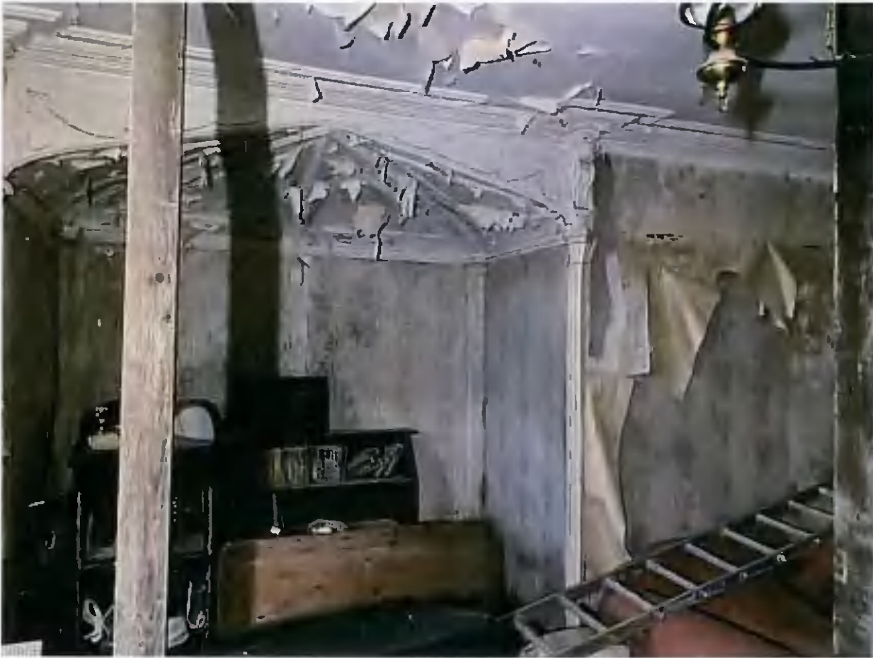
East Wall of North Room Behind Drum. Attractive apse moulding to be saved if possible (note timber props in foreground)
