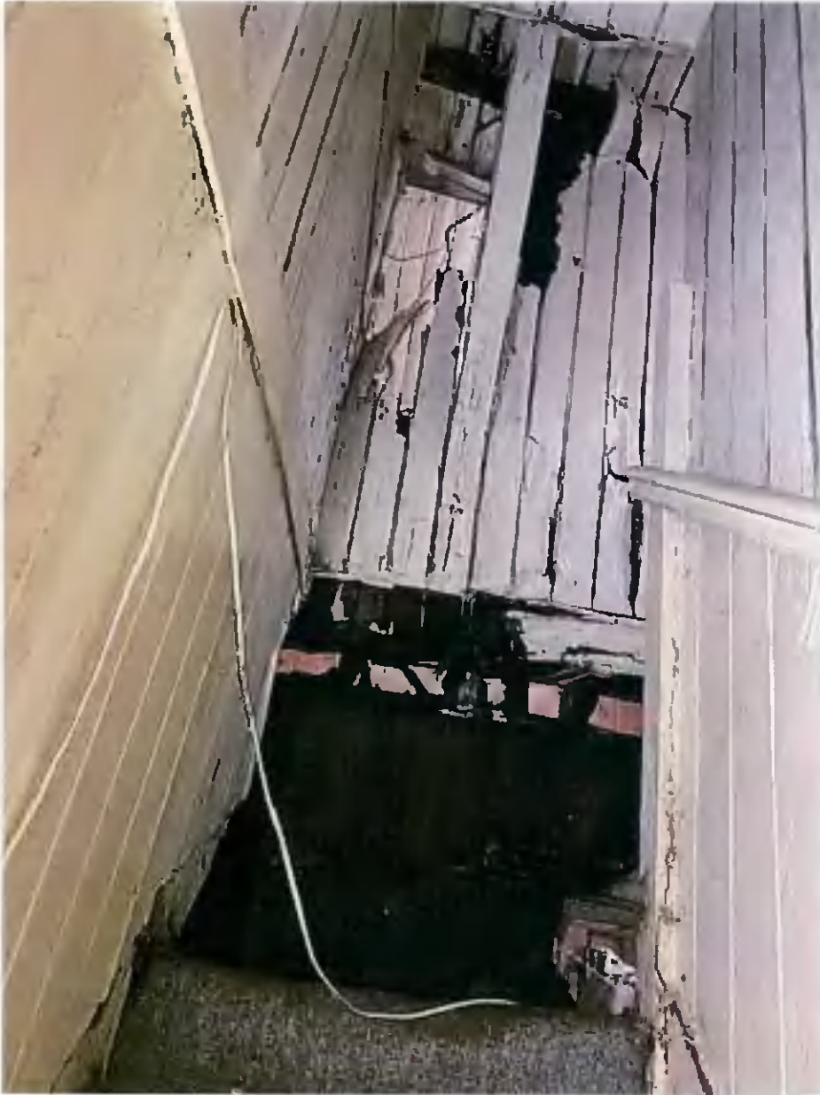
Detail of Internal Timber Lining
