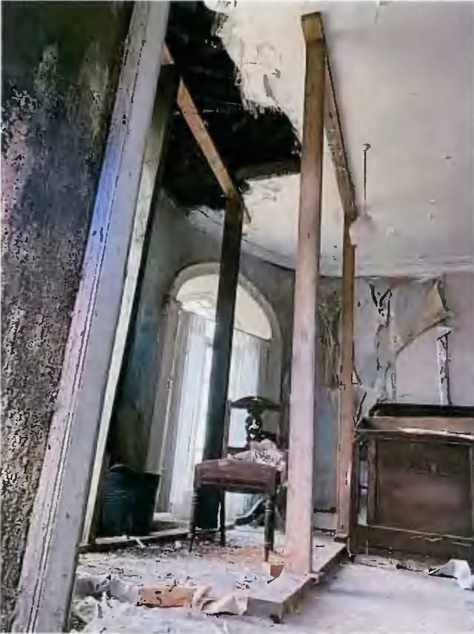
First Floor North Wall Behind Drum
