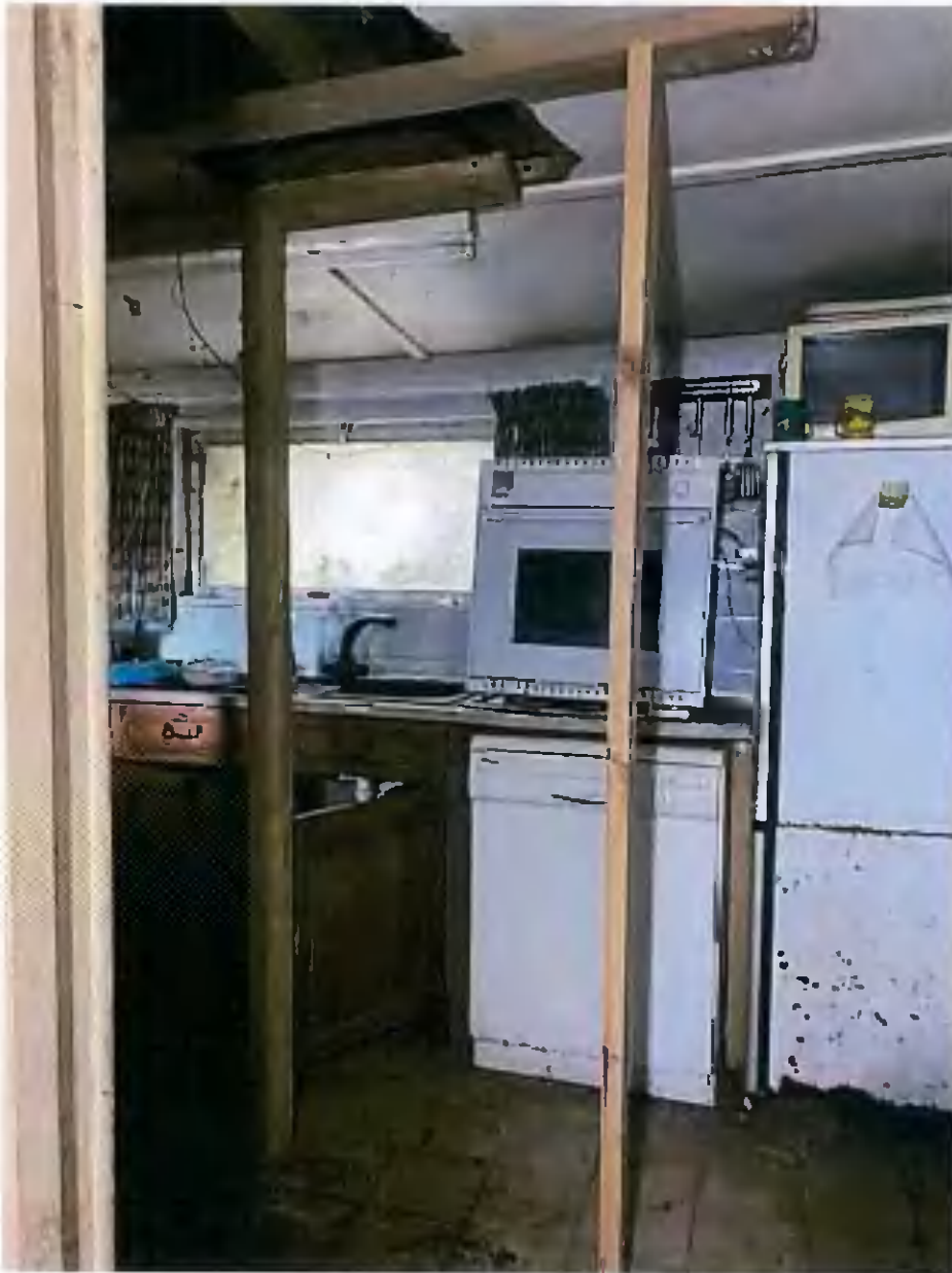
Central Rear Room
