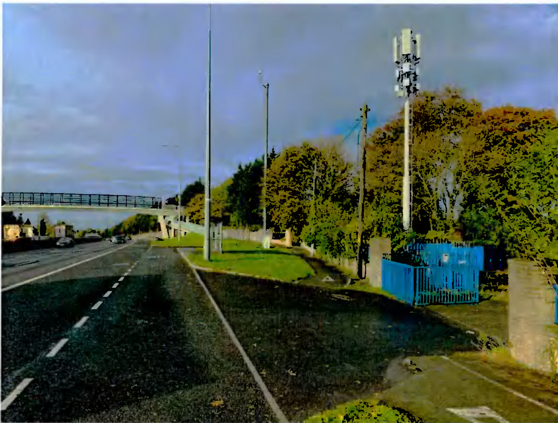
Figure 3: Aerial view of existing installation from the east
