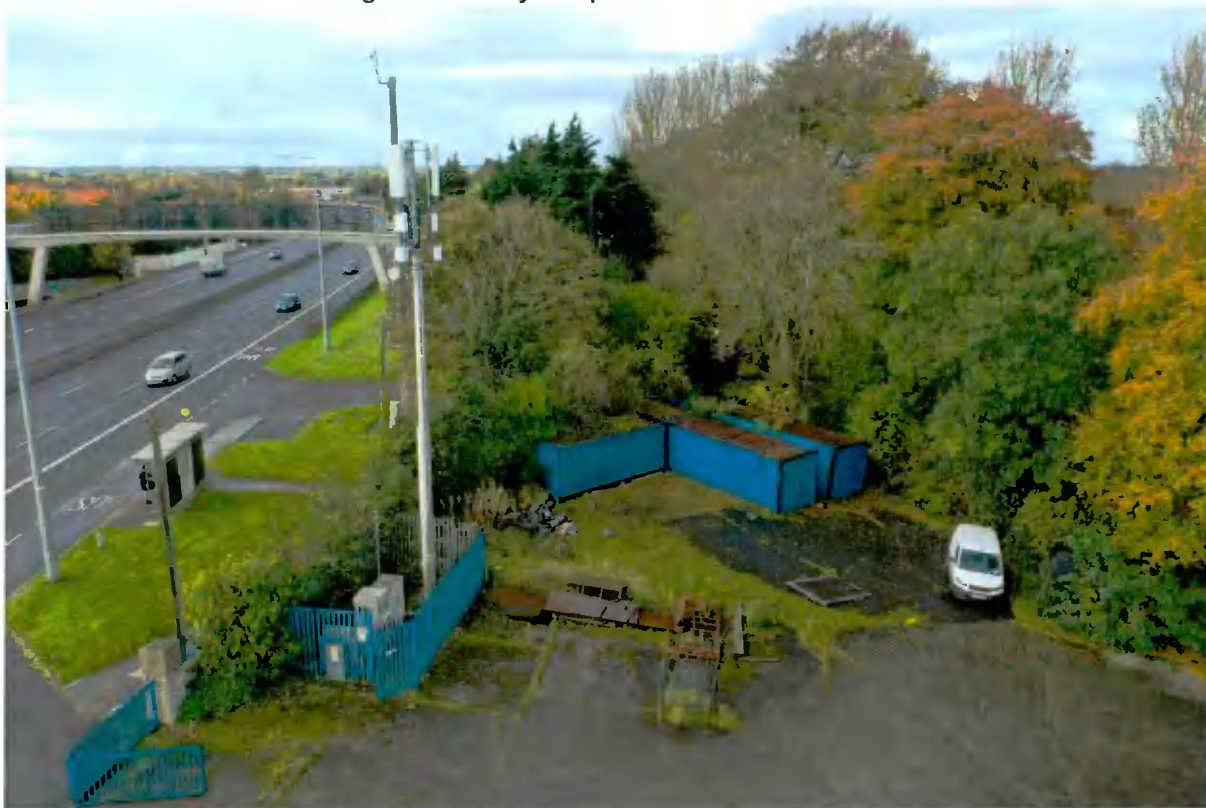
Figure 1: View of existing telecommunication installation
