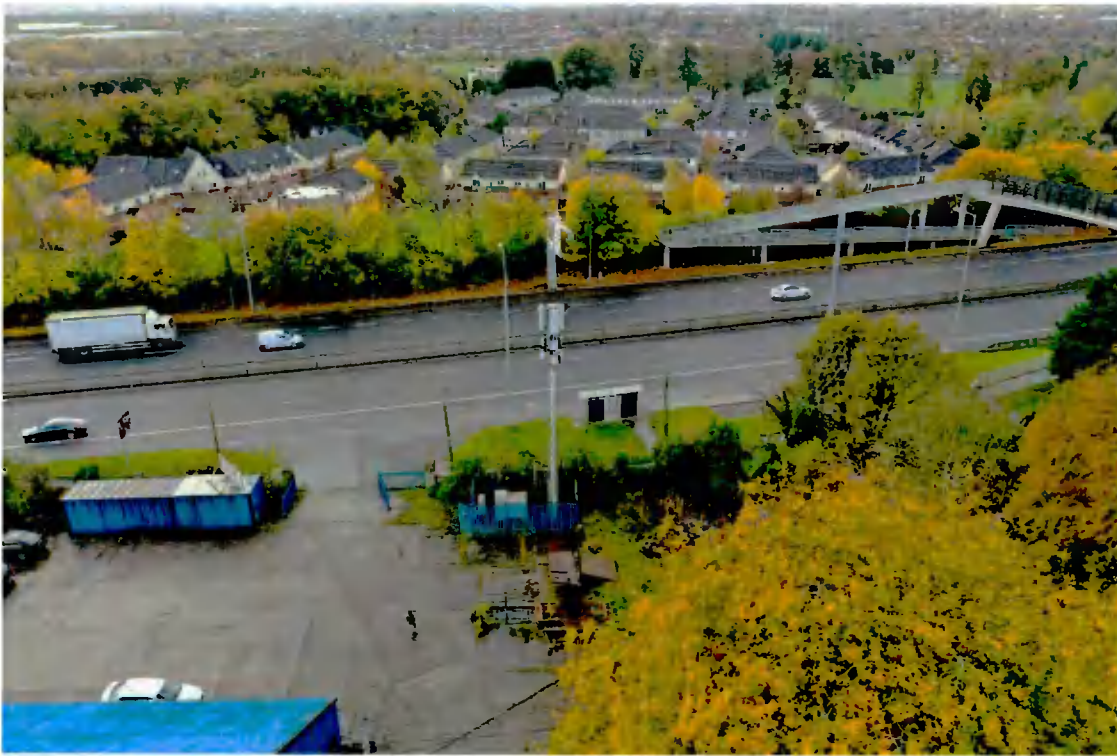
Figure 2: Aerial view of existing installation from the north
