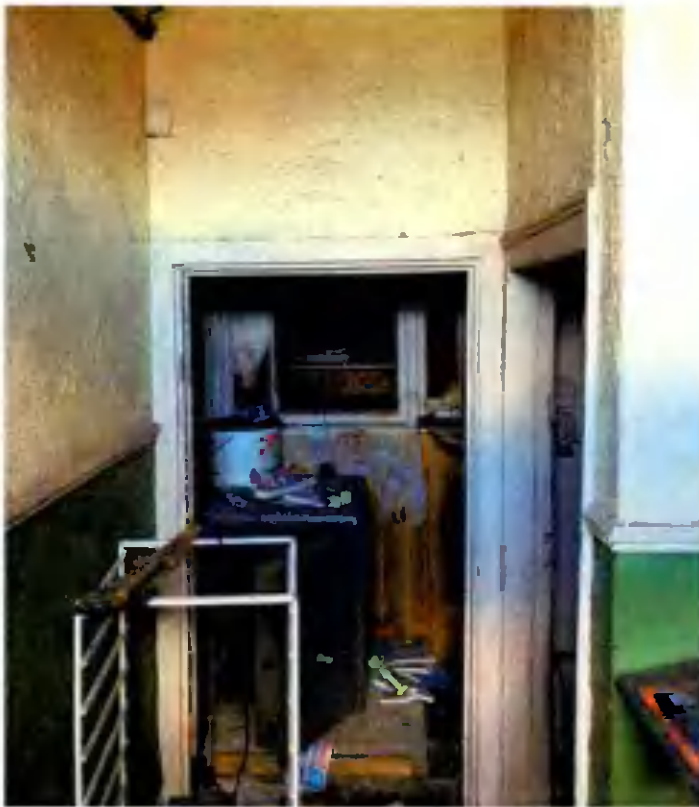
Internal view showing textured plaster at upper levels
