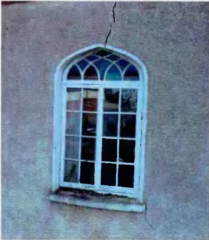
Typical gothic window with Y-tracery Note smooth render surround
