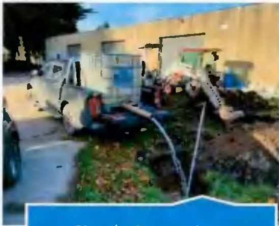
Site during testing - 19/11/2021
