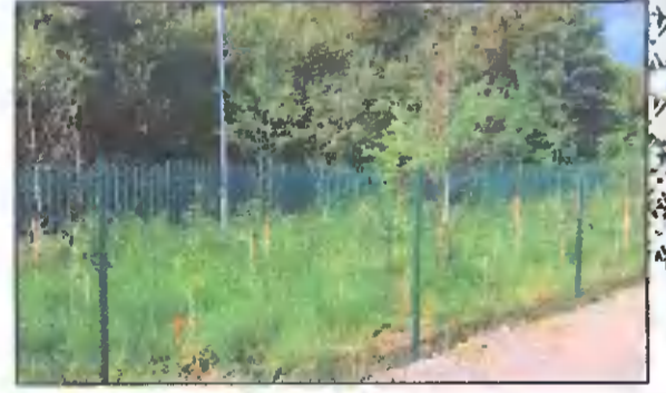
Boundary Type E New chainlink fence and buffer area of tree and woodland planting and fence as permitted under planning permission SD18A/0126
