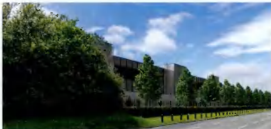
Picture 38: View of a proposed building from north-east
