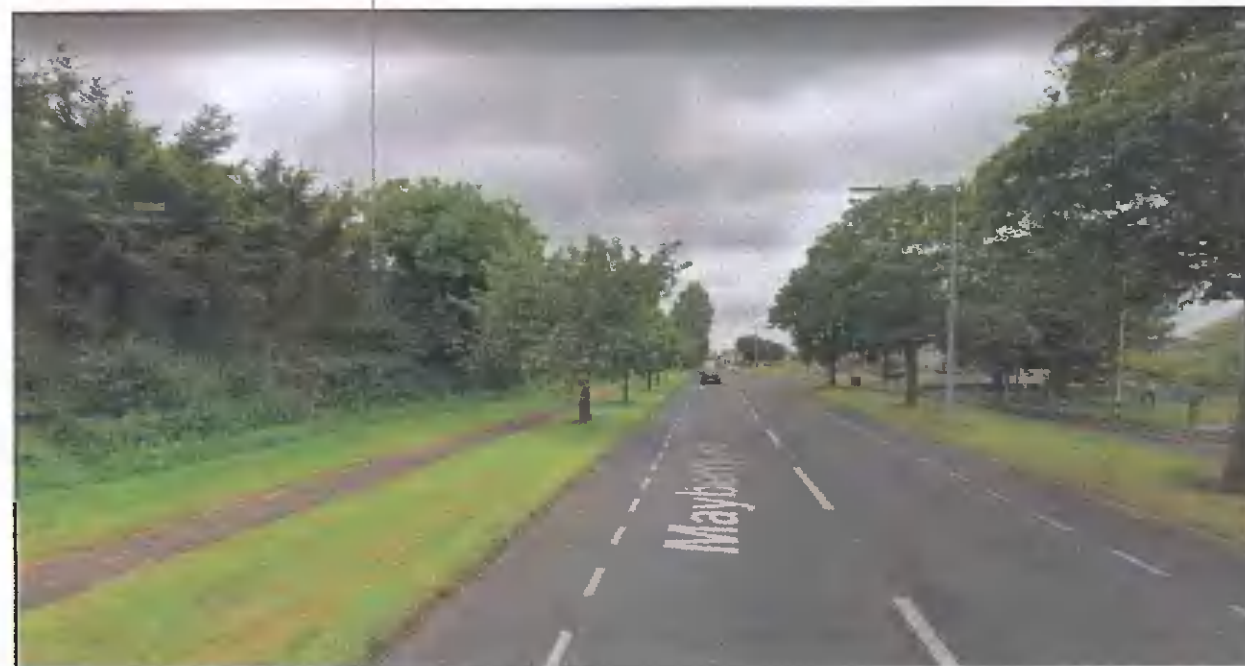
EXISTING VIEW WEST ON MAYBERRY ROAD
