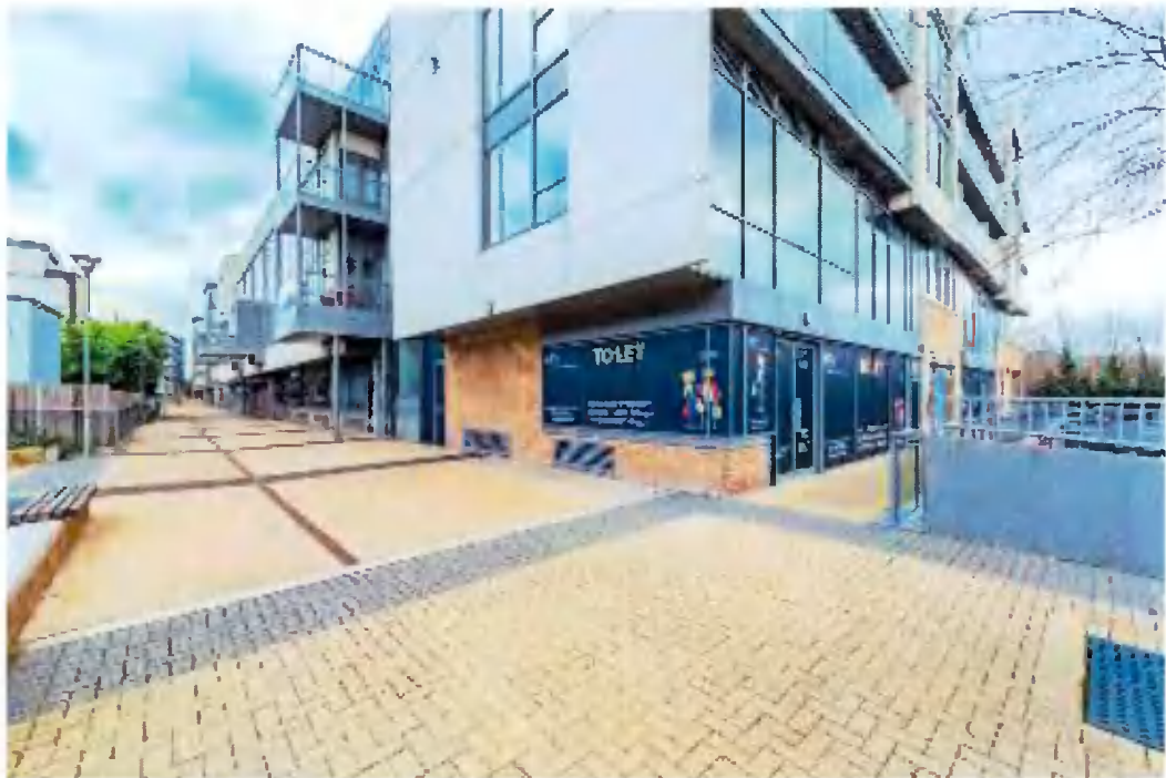
Figure 3: Photograph of Unit 3 and adjacent Pedestrian Street and Commercial Units
