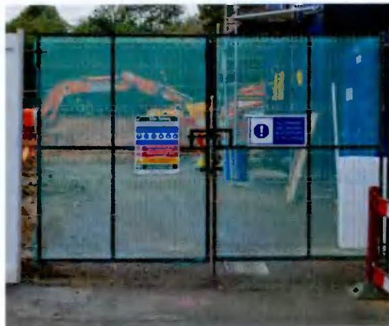
Figure 4 - Manned Security Gates
