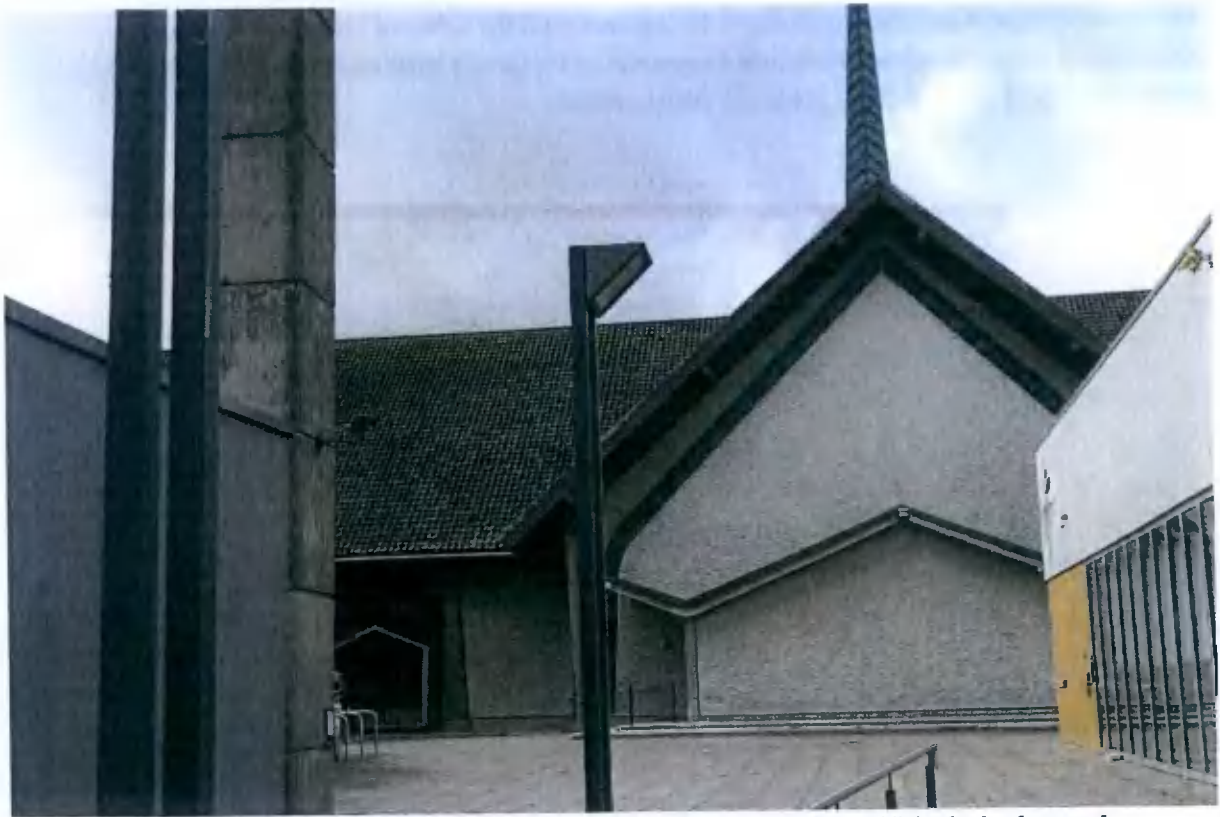
Fig. 3.15 Current chimney flue with Church of the Holy Spirit (RPS: 264) in the background.
