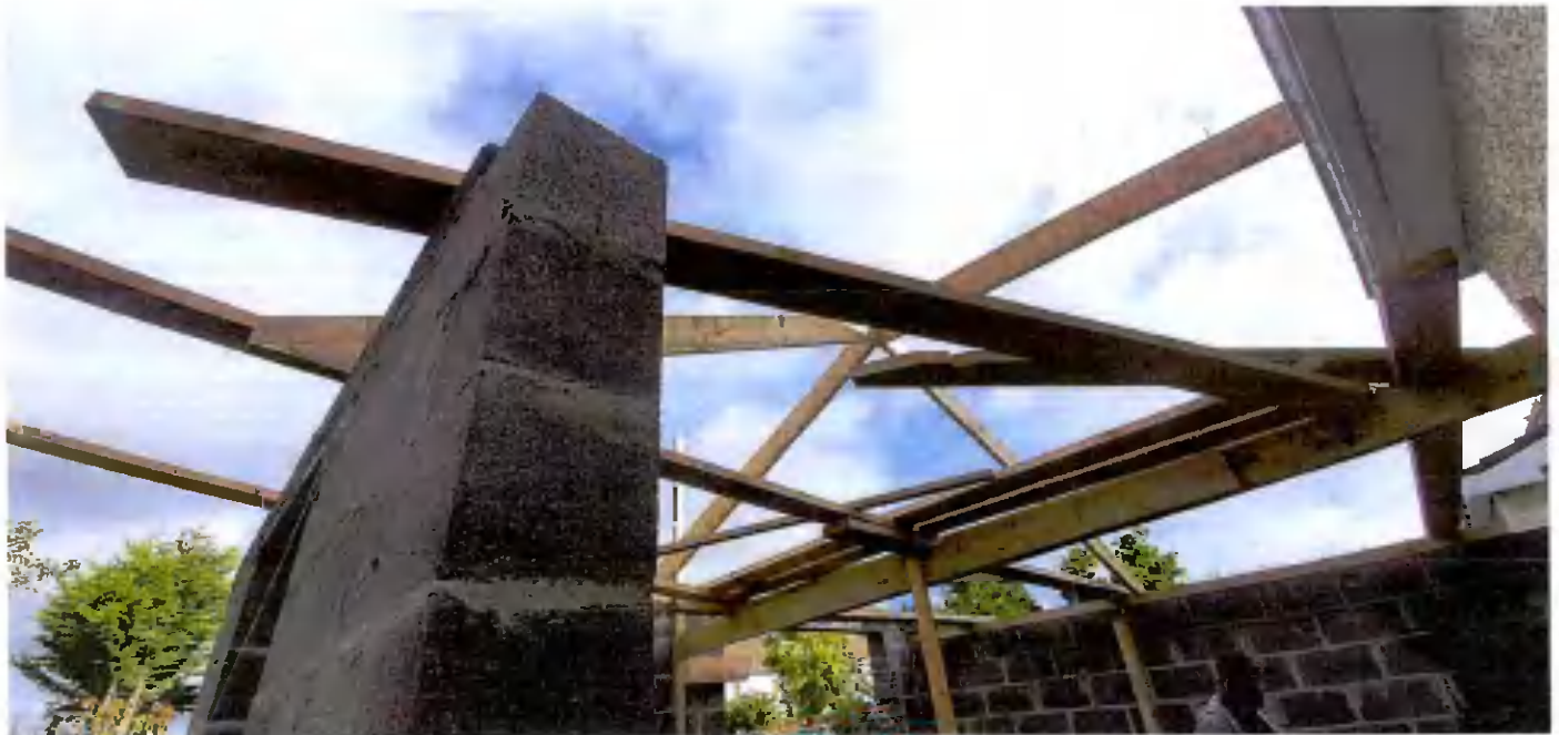
Figure No.4. Roof Structure and props
