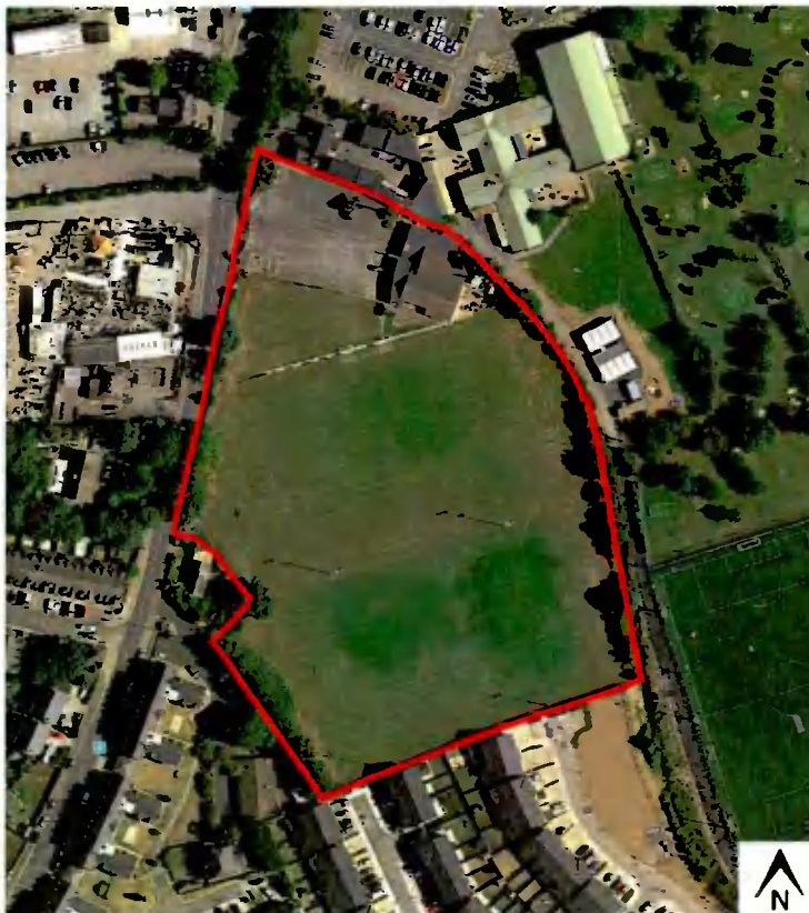
Fig. 1 – Aerial view of application site, outlined in red
