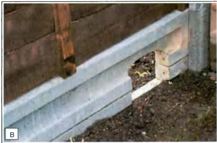
Figure 16. Examples of 'Hedgehog highways' that can maintain habitat connectivity for Hedgehogs in residential developments (Images: BHPS Guidance document).
