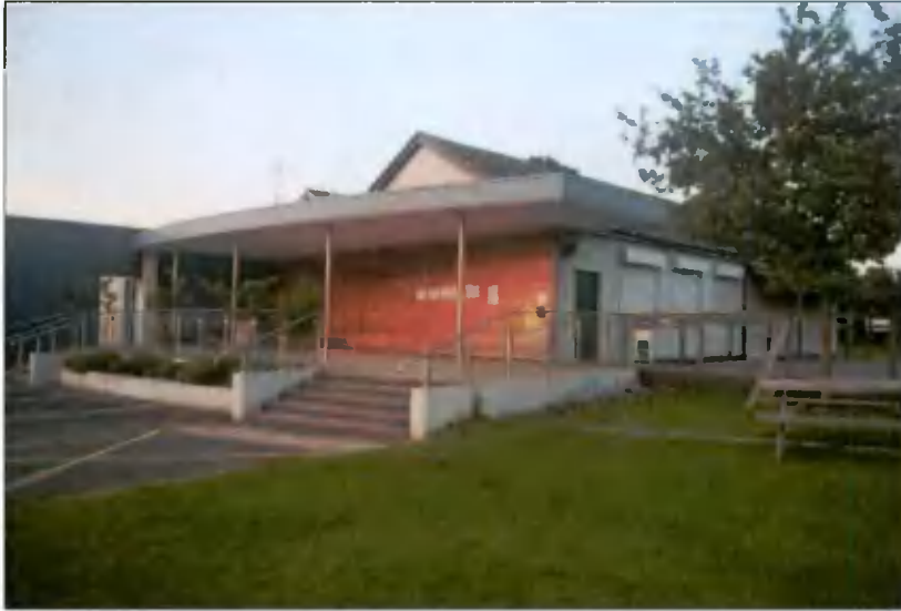
Plate 1 Existing Club House, Low bat roosting potential.
