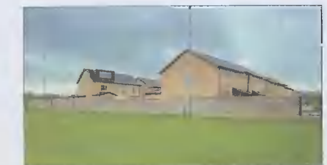
Existing Block Wall on Southern Boundary
