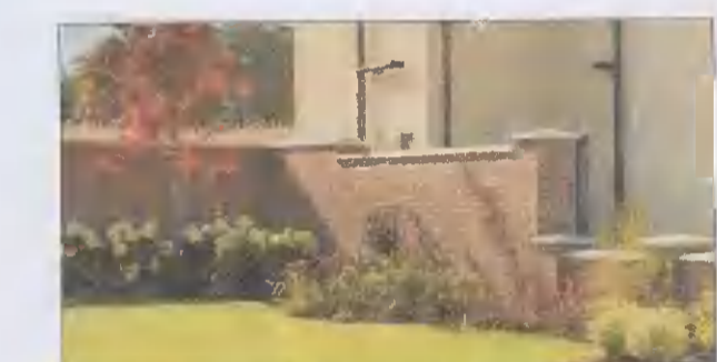
Concrete Block Wall with Brick Cladding
