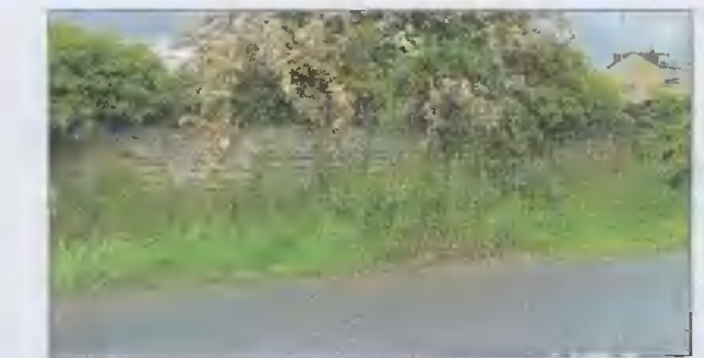
Existing Stone Wall Along Roadside
