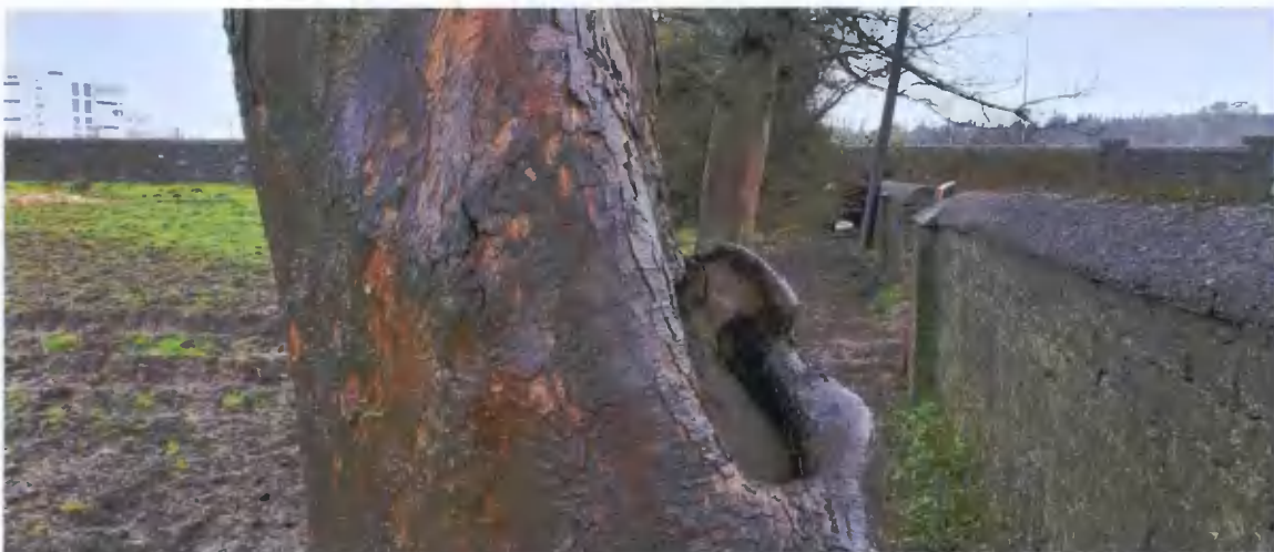
Figure 3-12 Large hole in Sycamore tree
