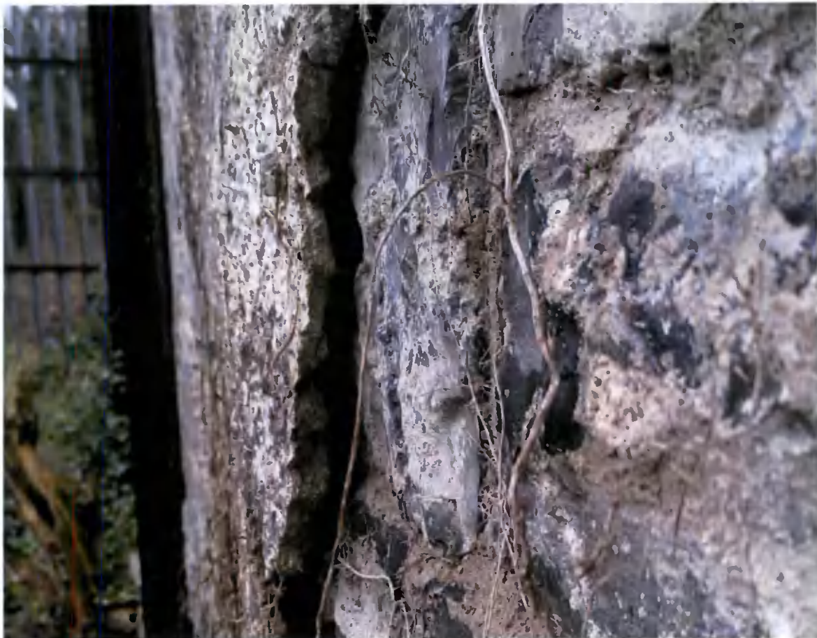
Figure 3-3 Space in between outer layer and wall
