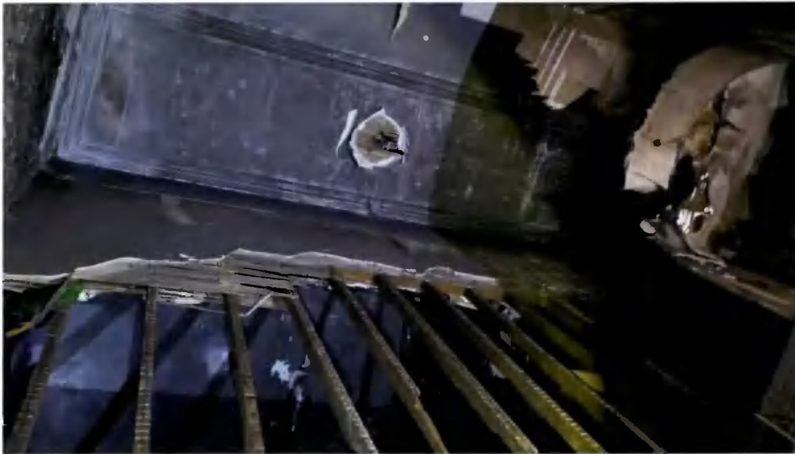
Figure 3-7 Ceiling Katharine Tynan House
