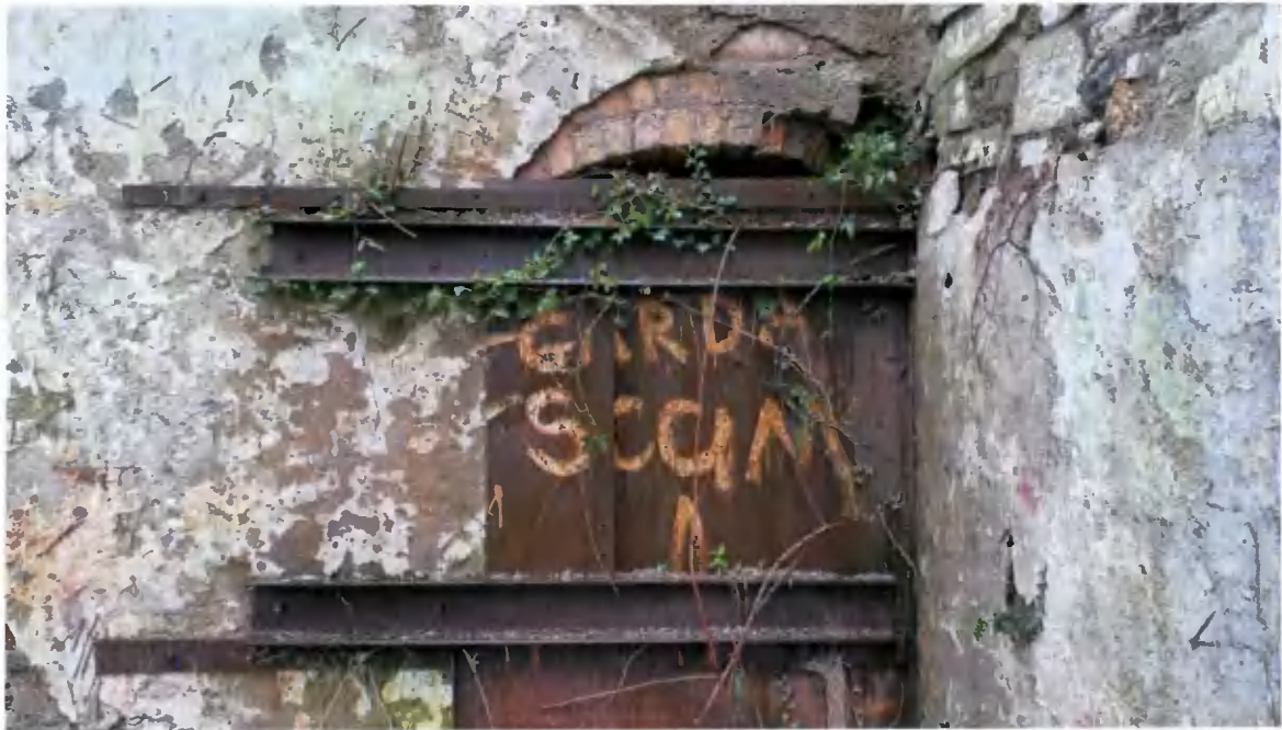
Figure 3-2 Potential entrance above door in corner (north facade)
