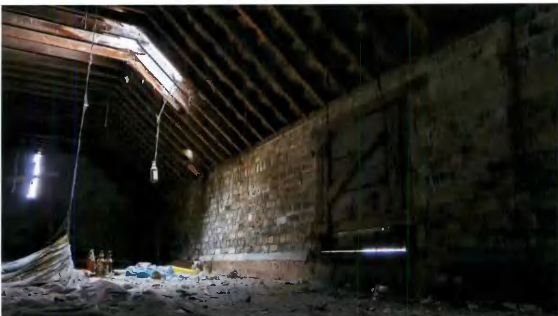
Figure 3-9 First floor of Newlands Villa
