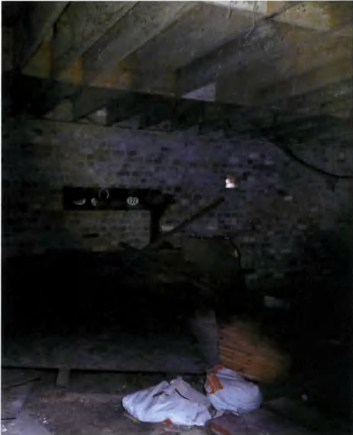
Figure 3-10 Ground floor of Newlands Villa
