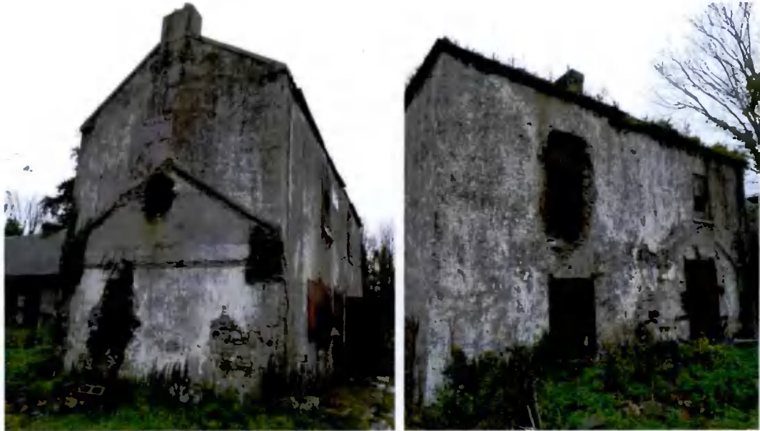
Figure 18: North and west sides of two-storey section Figure 19: South elevation
