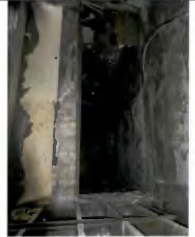
East elevation connecting corridor to Room 104
