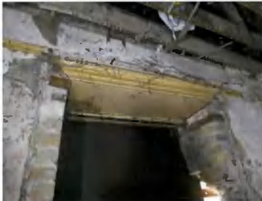
Figure 33: Timber lining to window in room G03
