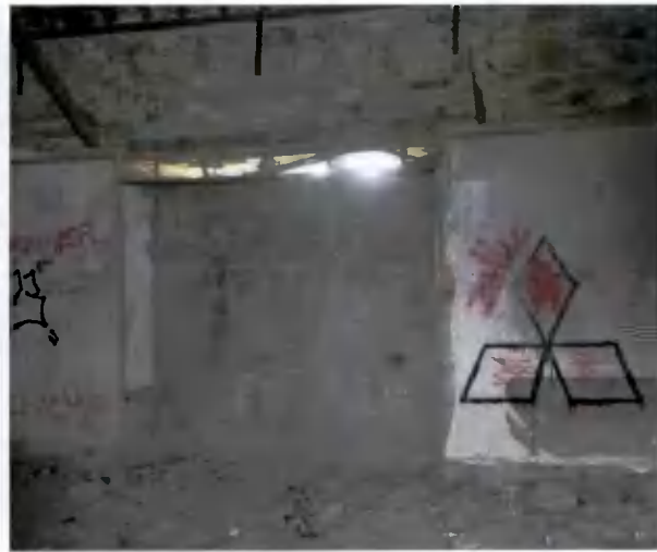
Figure 25: Missing lintel and weakened timber lintels above openings on north elevation
