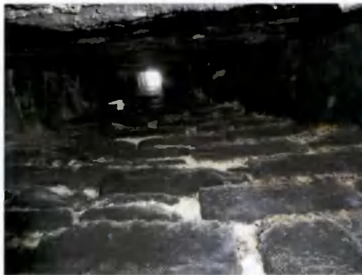
Figure 27: Flue in chimney in room G04
