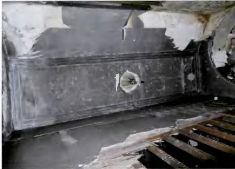
Figure 38: Ceiling above stair hall at first floor (room 102)
