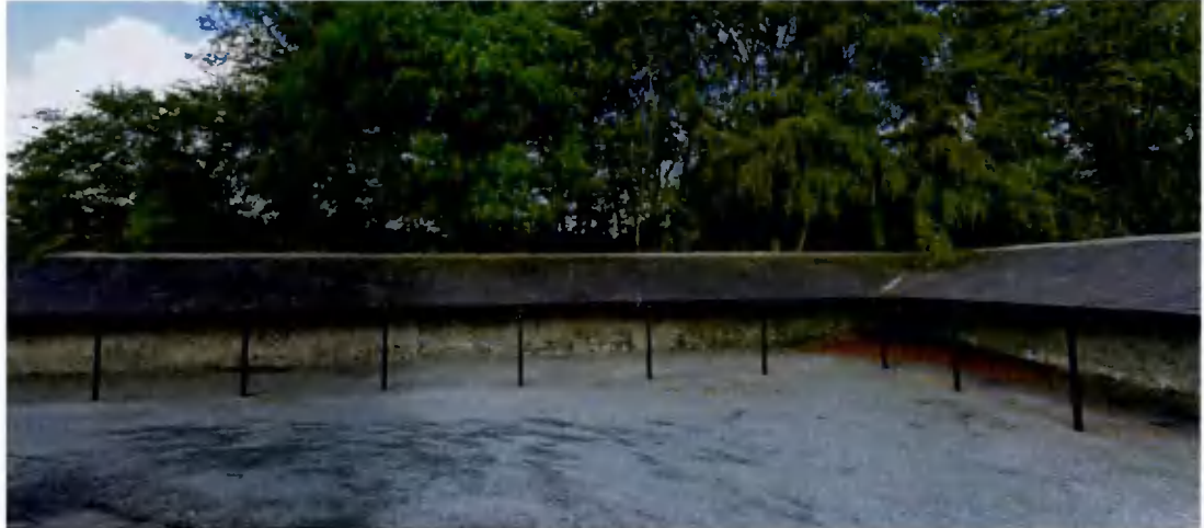
Figure 46: Historic roadside shelter at St.Paul's RC Church in Emo village, Co Laois
