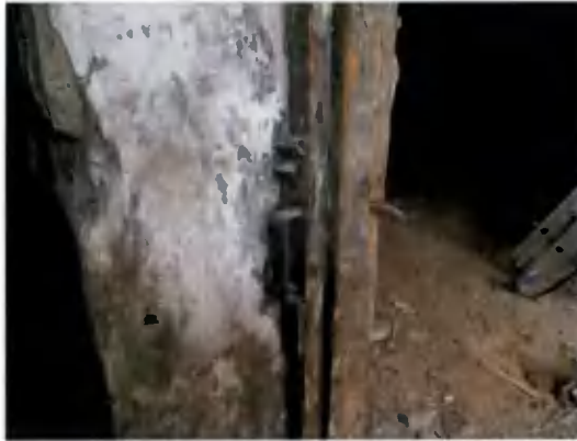
Figure 31: Door frame in room G01
