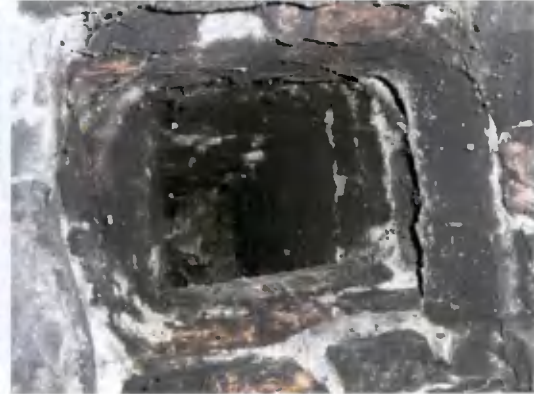
Figure 28: Flue in chimney in room G05
