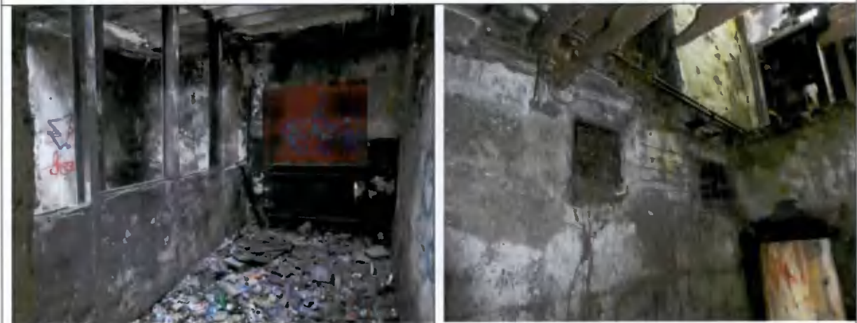
North and west elevations
