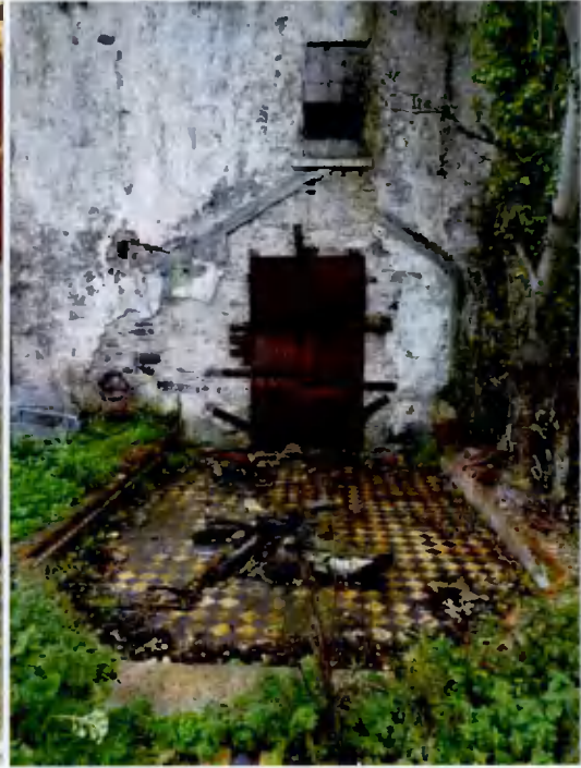
Figure 36: Former conservatory beside room DG03
