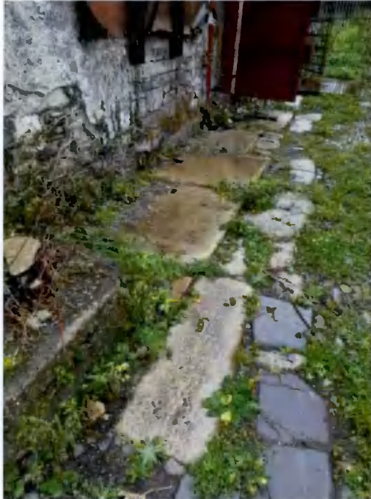
Figure 44: Stone paving at west side of house
