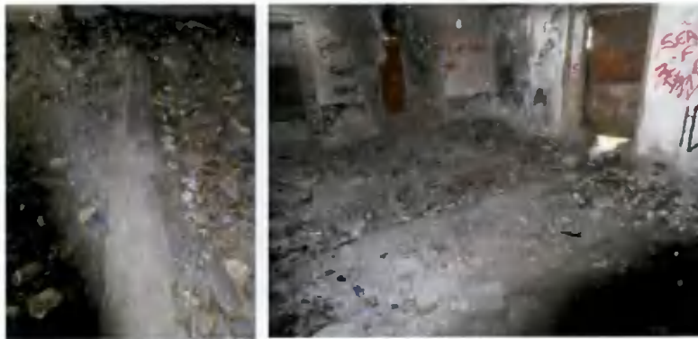
Figure 29: Remains of sleeper walls in Room G05
