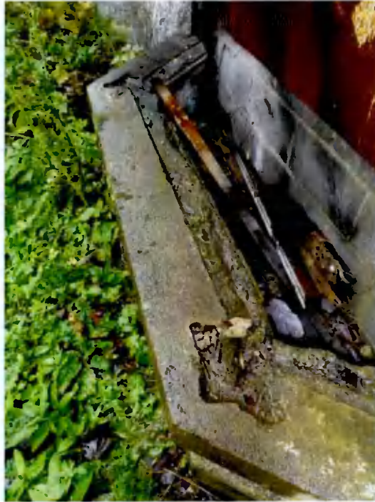
Figure 35: Bay window of room G05
