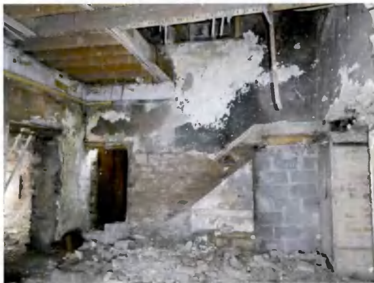
Figure 39: Wall marking of dog-leg stairs in hall (room G03)
