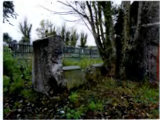
Figure 41: Garden wall at east gable
