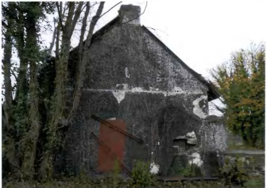
Figure 22: East elevation of single-storey section
