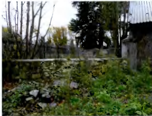
Figure 40: Garden wall at east gable
