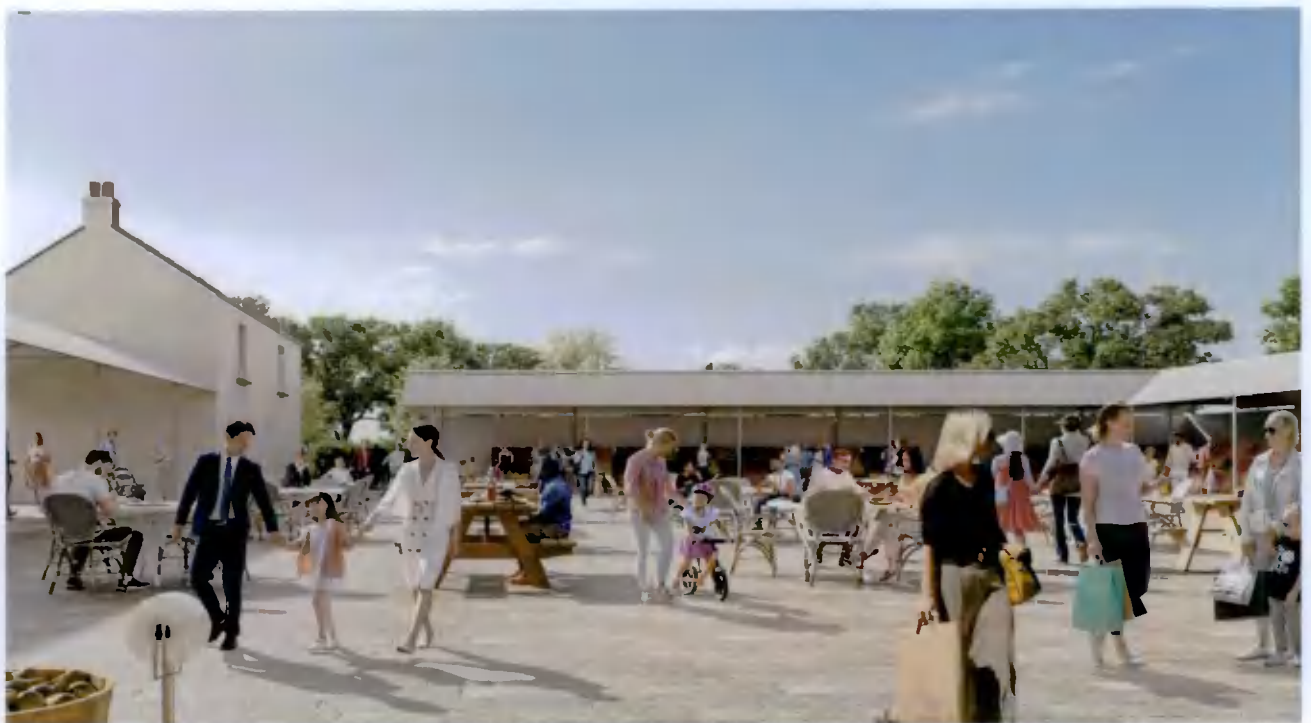
Figure Two: Concept CGI of Restored Courtyard at Katharine Tynan House (Source: Digital Dimensions, 2021).
