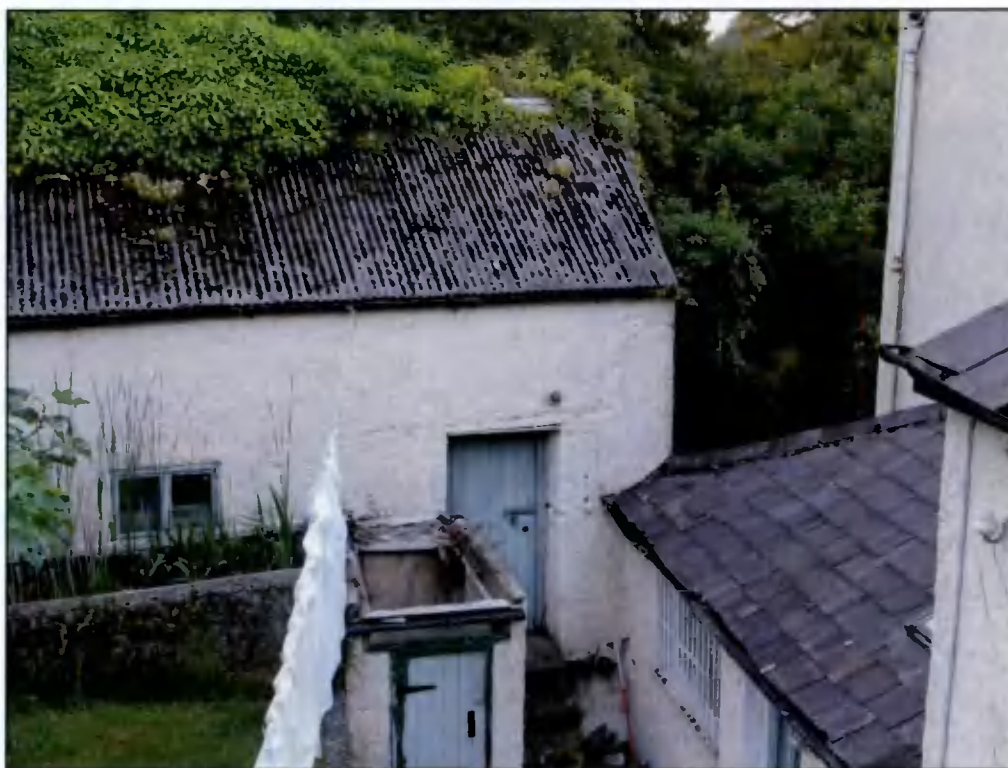
Figure 6: Outbuildings/sheds adjacent to Palmyra House
