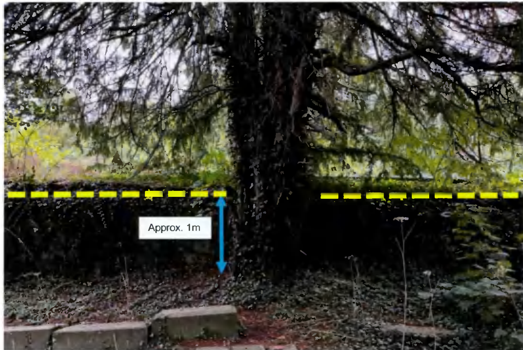
Photo 1: View of the main stem of the mature A Category yew (T643) tree from within the graveyard. The yellow line indicates the top of the wall which is also the top of the adjacent shed to be demolished. This is a retaining wall and is restricting root growth into the Application Site.
