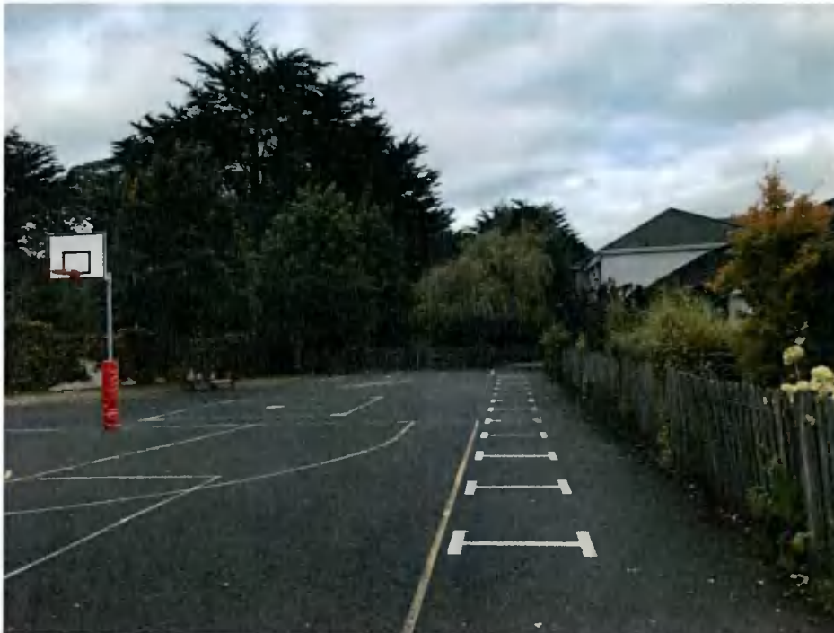
Figure 2; Looking towards the proposed construction area
