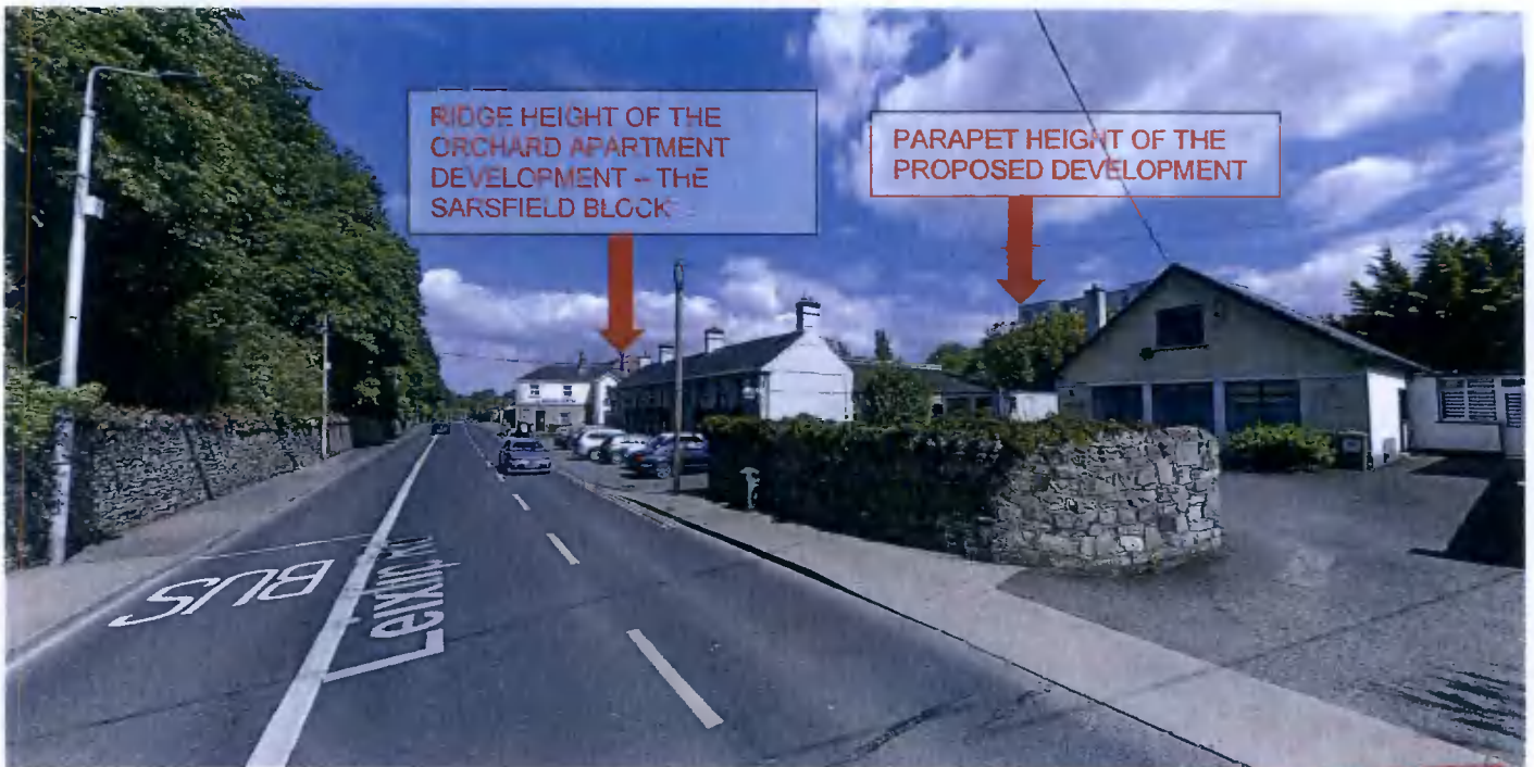
View looking back along Leixlip Road with The Orchard Apartment block known as 'The Braeburn' in the background and the proposed development
