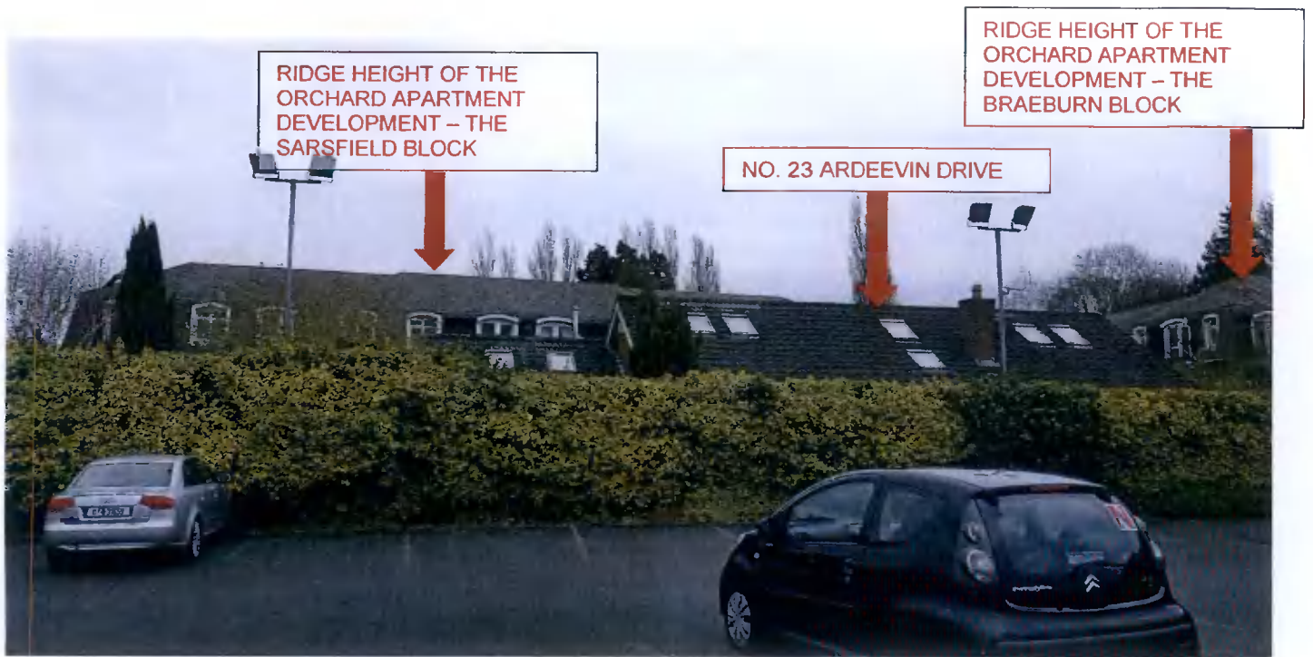
View from within subject site looking towards No. 23 Ardeevin Drive and The Orchard Apartment Development (3-storey with pitched roof)
