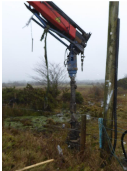
FIGURE 3. UTILITY TRUCK MOUNTED AUGER EXCAVATING HOLE FOR UTILITY POLE
