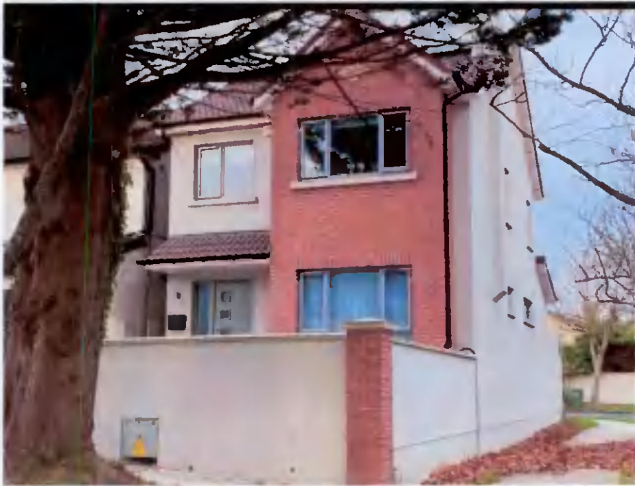
8a Rossmore Grove SD18A/0117 —example of elimination of 1 side entrance on boundary side and maintain functioning side entrance on opposite side (as shown in our proposal), and window positioning on boundary wall
