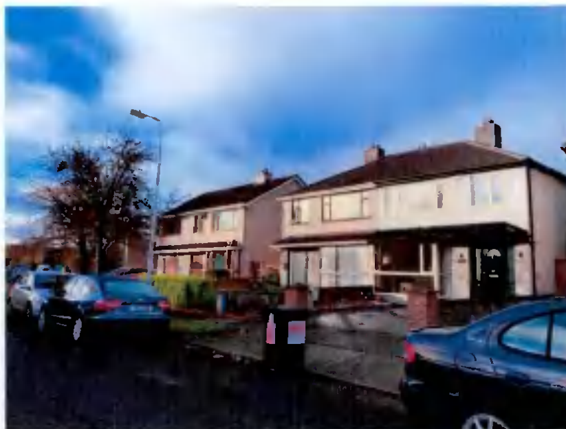
440 Orwell Park Green example of pitched roof gable to gable at end of row of hip roofs.
