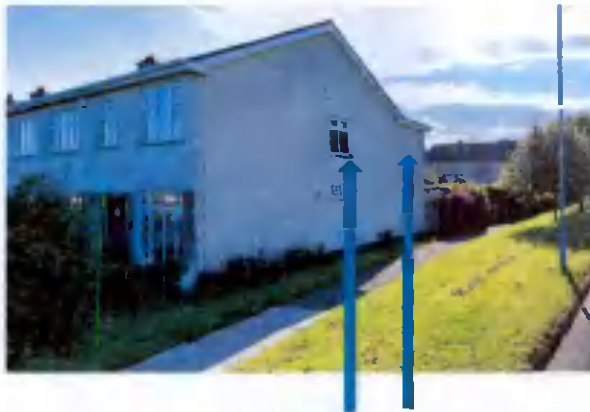
1 Osprey drive — window in party wall with public space & and rear building line has moved beyond established building line , similar to what is proposed in our development -Granted approval
