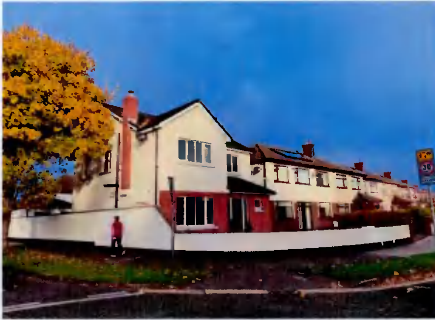
1A Domville road example of pitched roof gable to gable , at end of row of hip roofs.
