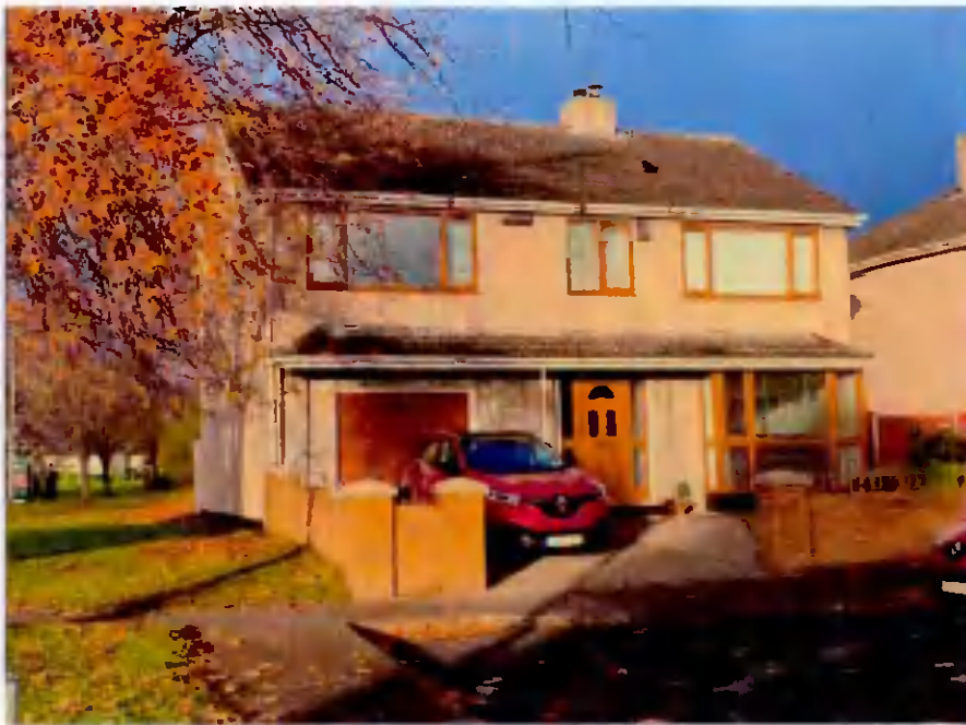
440 Orwell Park green — example of pitched roof gable to gable , at end of row of hip roofs & example of elimination of 1 side entrance on boundary side and maintain functioning side entrance on opposite side (as shown in our proposal)
