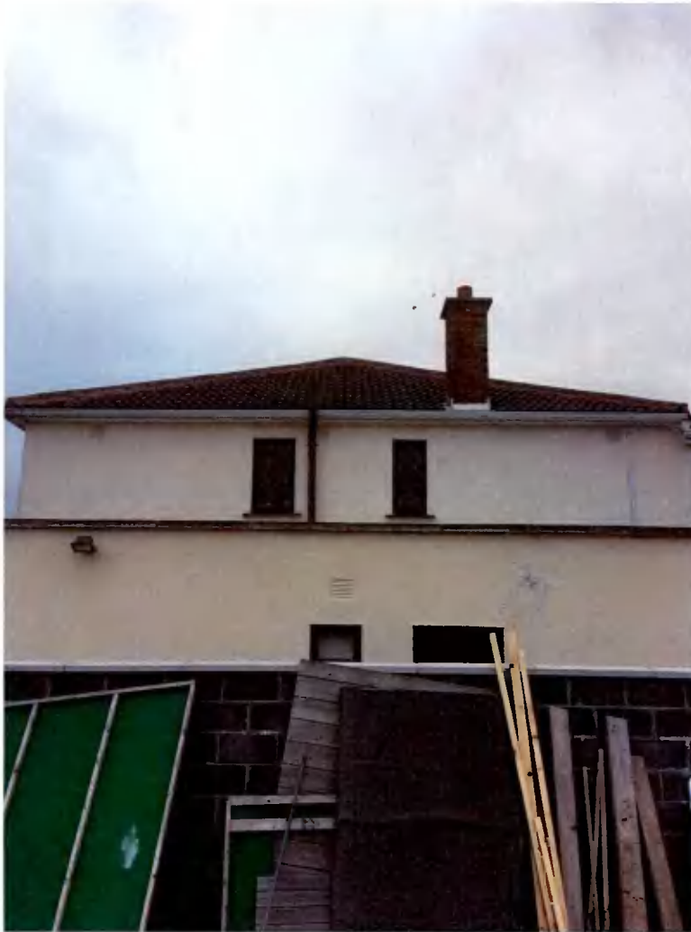
Image 04 – Photograph showing existing side elevation with no windows to habitable rooms
