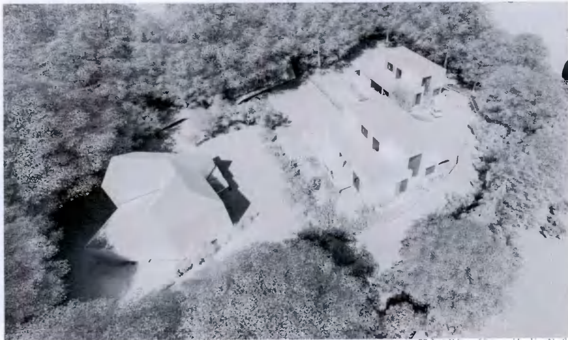
02 Aerial View of Proposal Looking North
