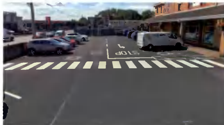
Fig. 5: Areas outlined as pub car parking not marked as such in within the shopping centre car park (1)
