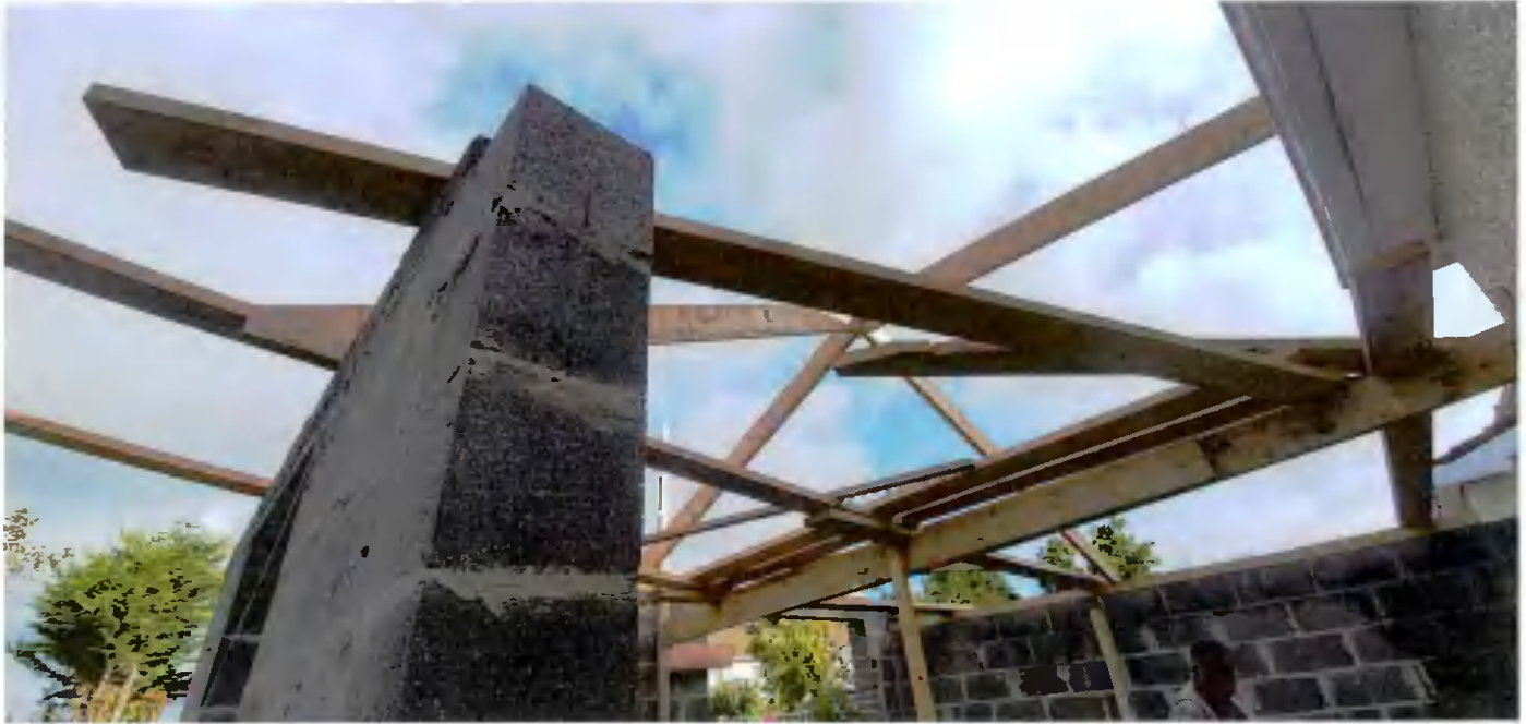
Figure No.4. Roof Structure and props
