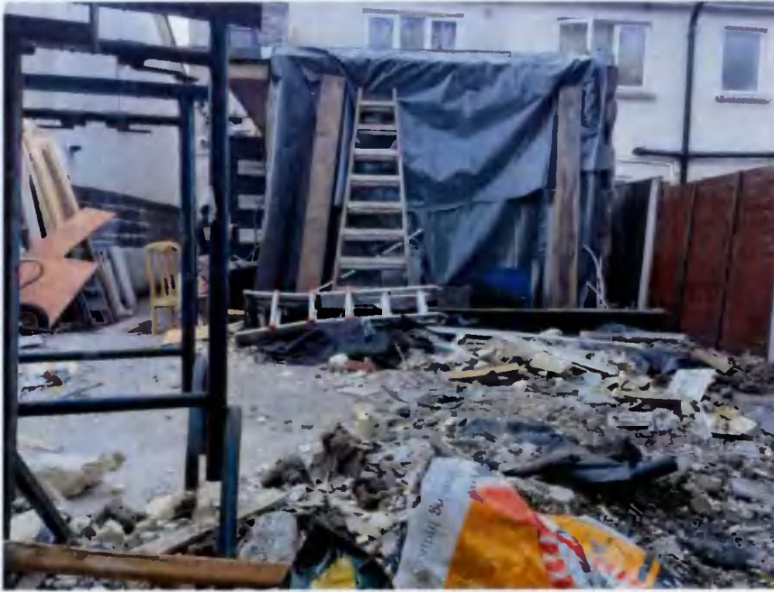
Fig 3. Storey-and-half section of existing Extension taken down
