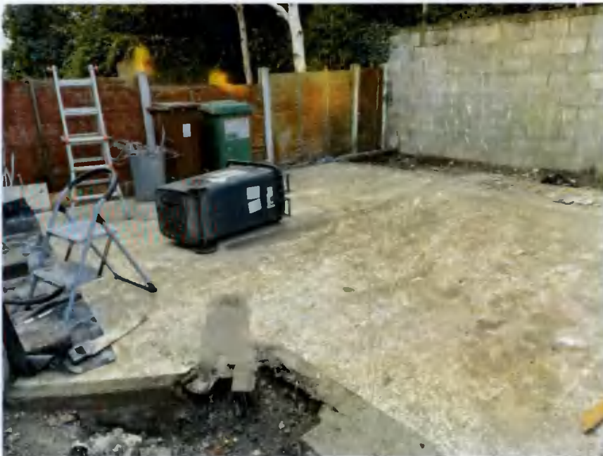
Fig 4. Debris removed from the back of Site.
