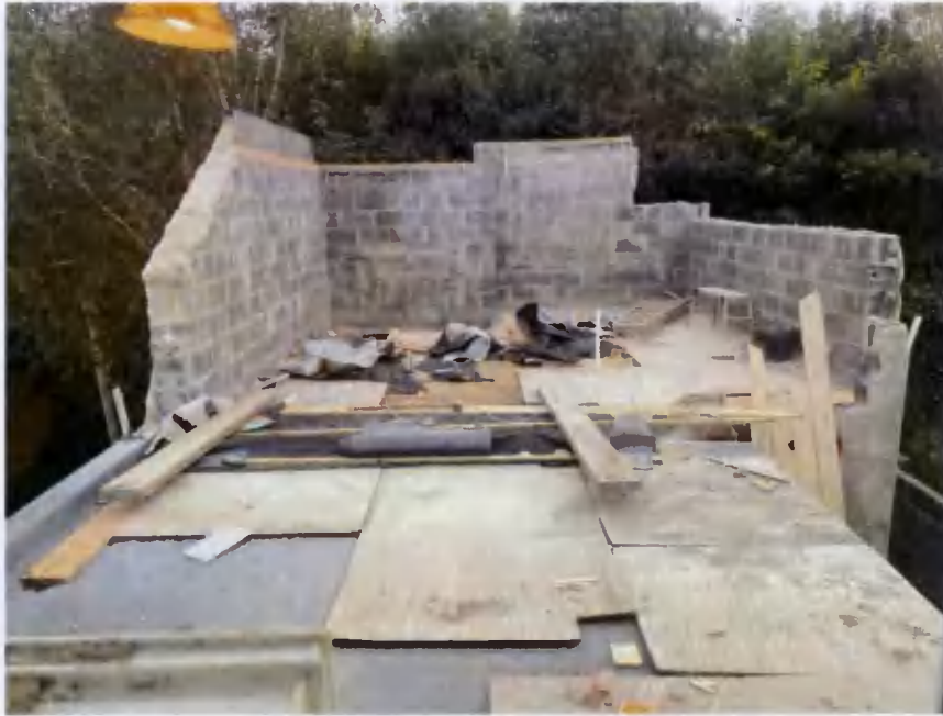
Fig 1. Pitched Roof and walls to non-habitable Attic taken down
