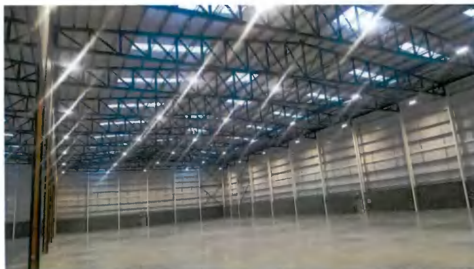
Typical clear open space warehousing facility
