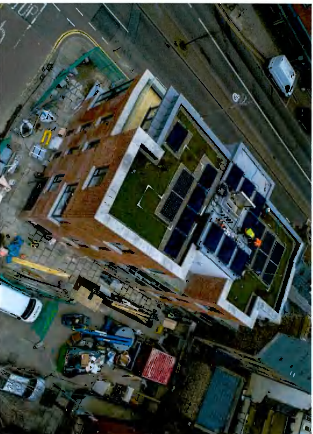
New Street South Development - PMVT - FKP completed project 2021
