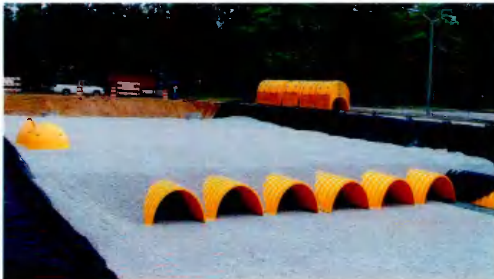
Figure 9 - Typical Cellular Storage (Stormtech) Installation
