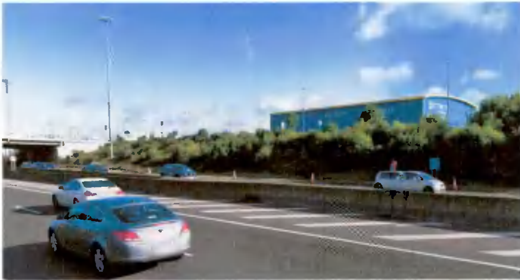
Fig 5.5 U Store It unit at Ballymount, seen from the M50
