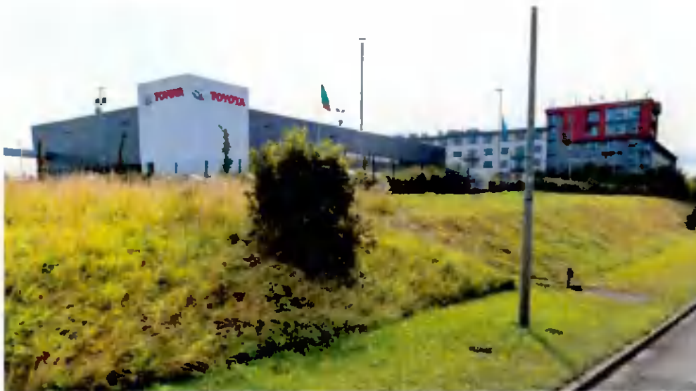
Fig 5.1 View of Toyota Garage and Hotel from N4
