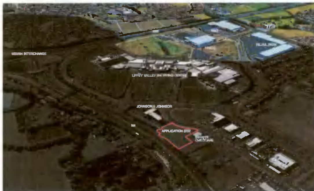
Fig 2.1 Site Location, Aerial View
