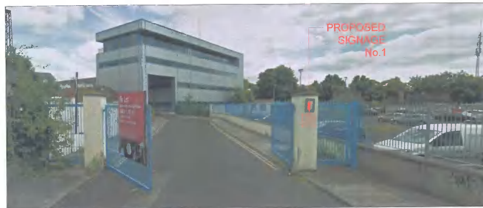
Photographs of existing (with intended location) Scale 1:10
