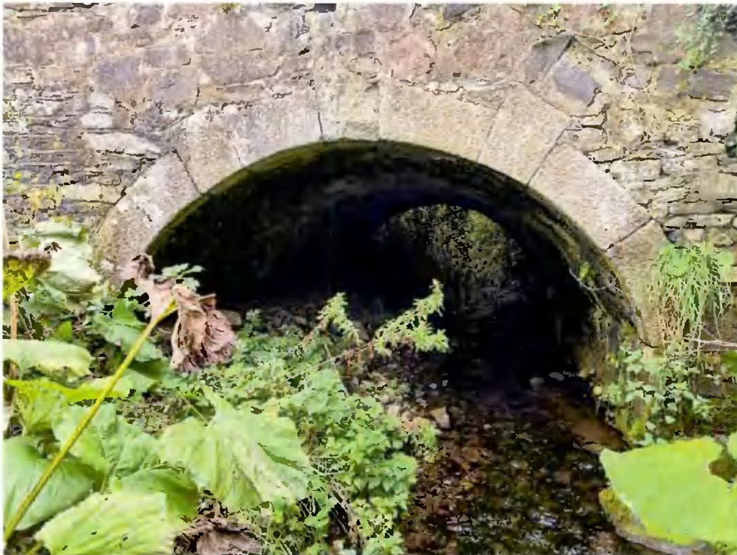
Plate 6. Photo of L6018 – Local Road Bridge traversing the Camac Stream to the north-east of the site.
