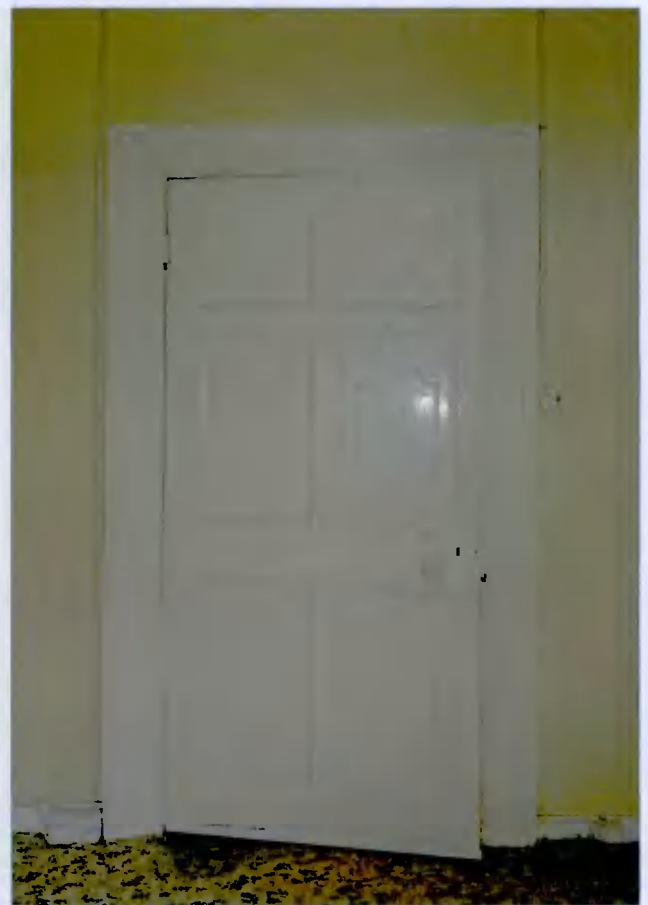
Inside of door to the south east upper room
