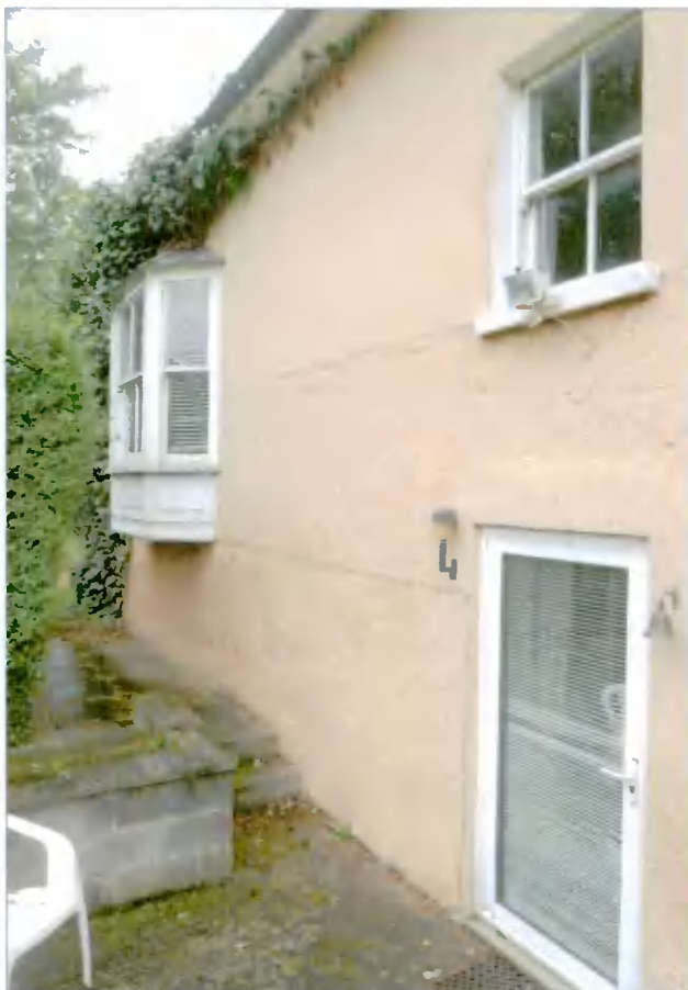
South side of house. A new bay window is proposed at ground level, replacing the door seen on the right.
