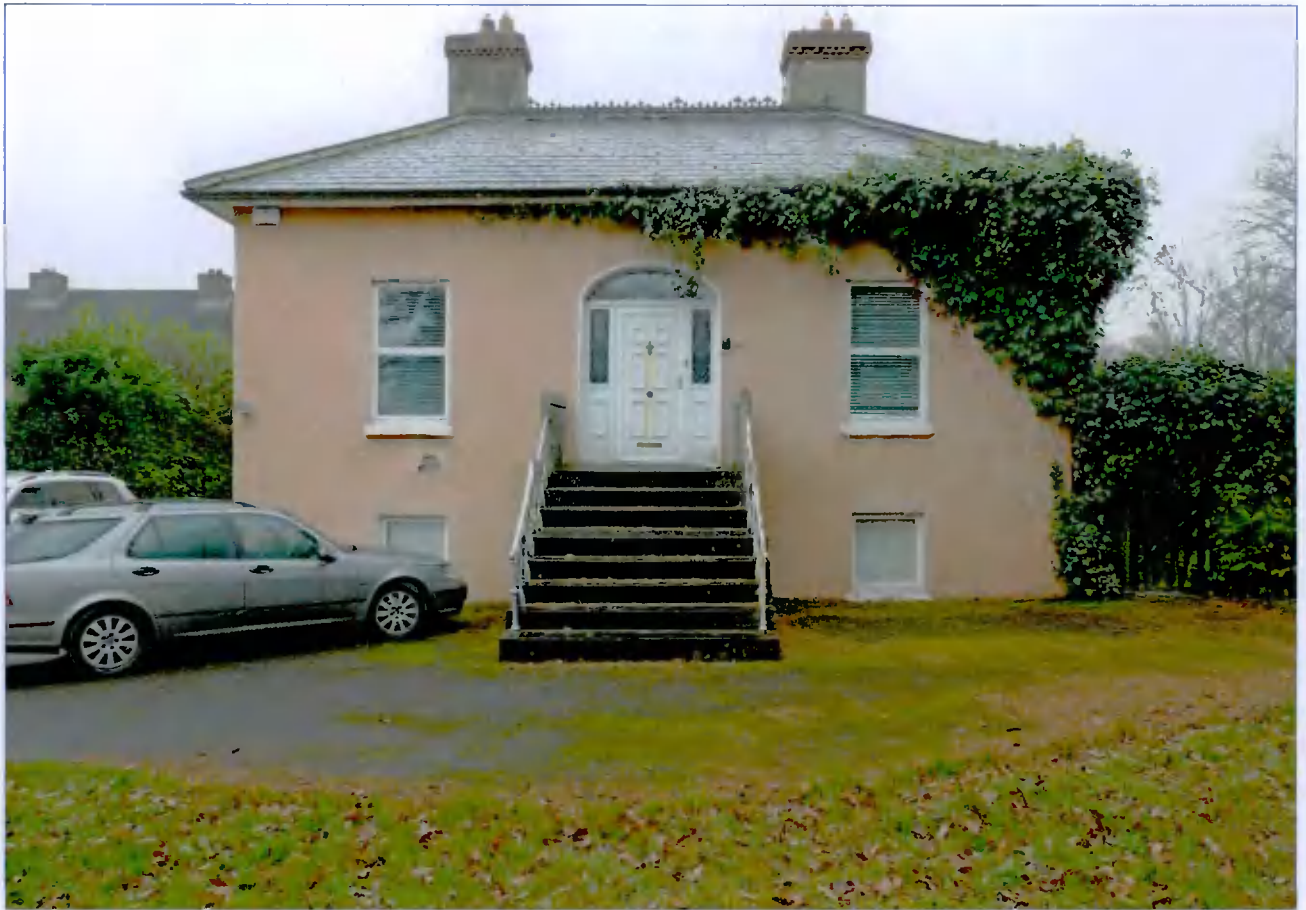
Front (west) facade. It is proposed to replace the existing uPVC windows with timber 1-over-1 up-and-down sash windows detailed appropriately and to replace the modern door and doorcase with a timber door and doorcase of a design and detail appropriate to the period of the house
