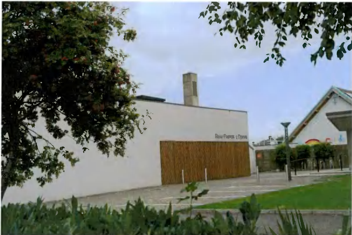
Fig. 3.14 Height of the existing chimney flue in relation to the pastoral and youth centres.
