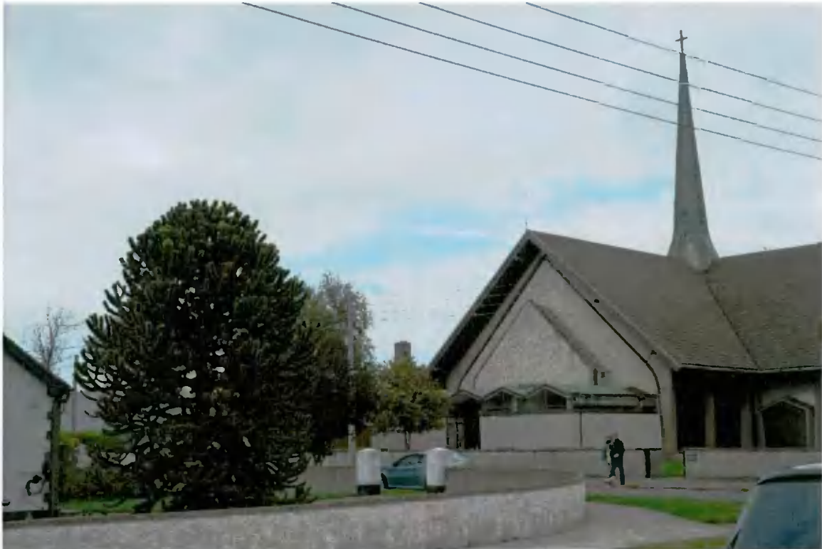
Fig. 3.9 Church of the Holy Spirit (RPS: 264) brings historic character and distinctive landmark to the visual environment.
