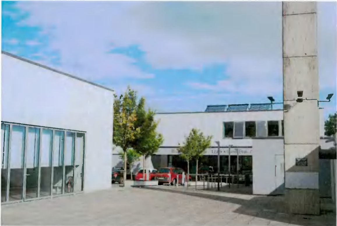
Fig. 3.13 Location of proposed site. Proposal to replace existing chimney flue. View looking north with library in the background and pastoral centre to the left.
