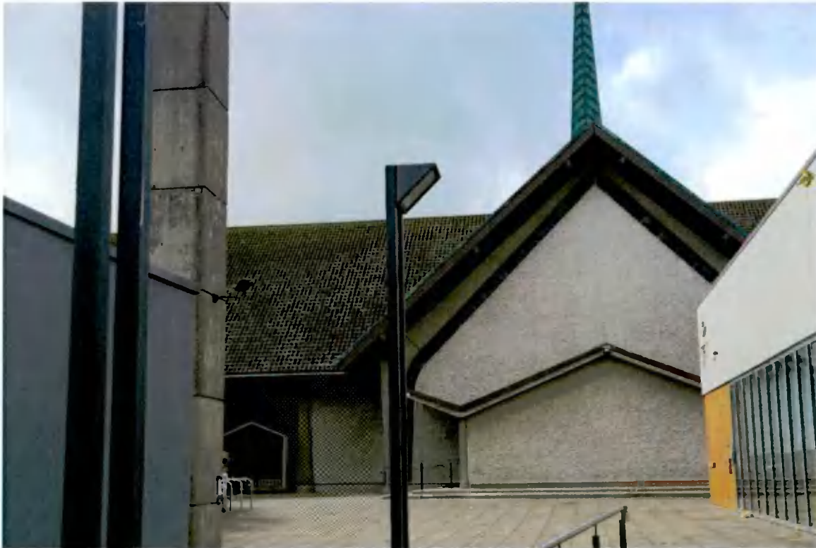
Fig. 3.15 Current chimney flue with Church of the Holy Spirit (RPS: 264) in the background.
