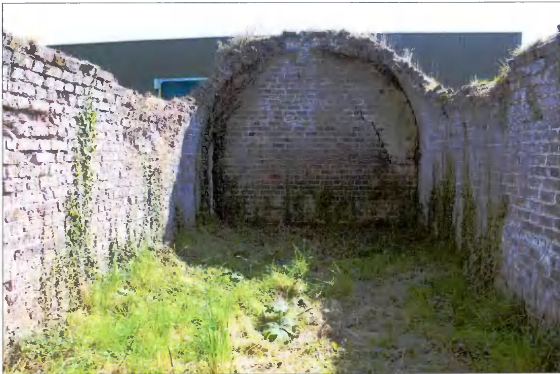
Plate 4: Interior of former gunpowder store from doorway at north-west gable end.
