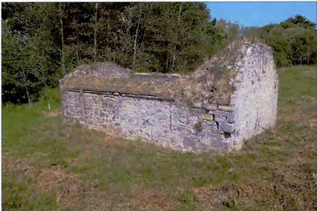
Plate 2: South-west side elevation and south-east gable end.
