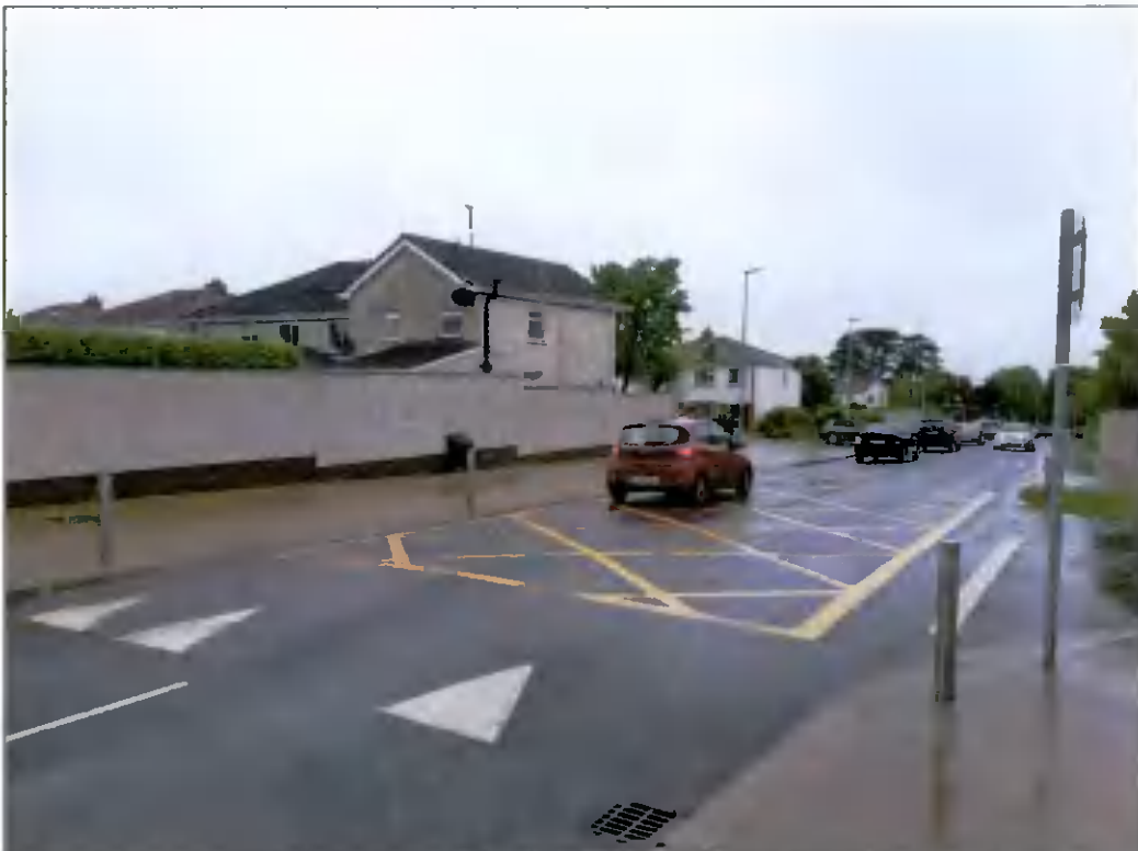
View of side & rear elevation as existing from Scholarstown Rd. looking north.
