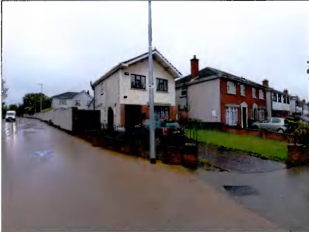
View of 1, Beverly Drive as existing
