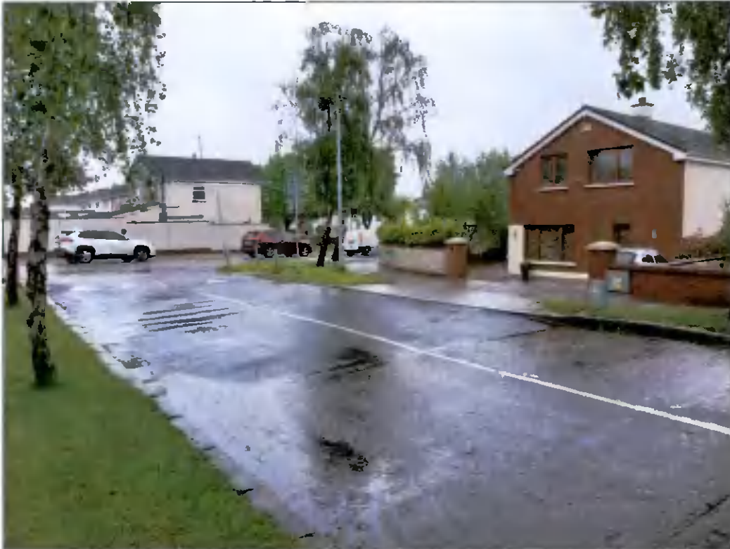
View of existing side elevation, seen from The Rookery development.
