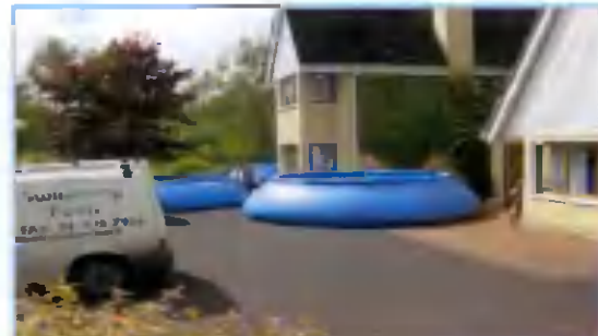
Photos show temporary above ground pools to store water when Filling or carrying out repairs
