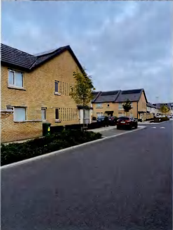
Managed Landscaped gable strips at St. Helens Phase 2, Adamstown
