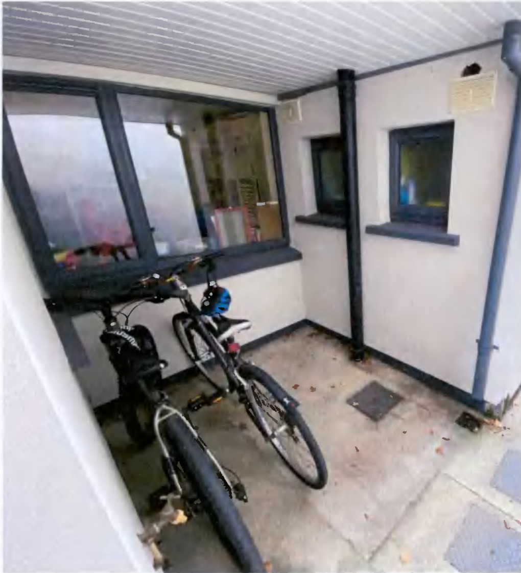
Figure 2. Bicycle storage area
