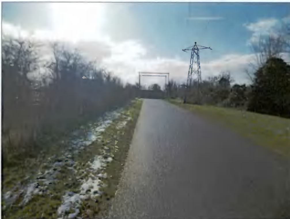
Plate 2: Existing road between WTP sites – dosing line is proposed to left of frame behind fenceline/treeline. Facing S.
