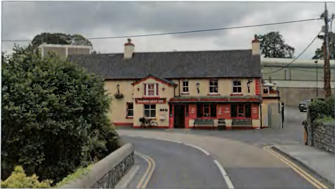
Plate 5: Salmon Leap Public Inn (RPS: 009) with existing WTP infrastructure visible to rear.
