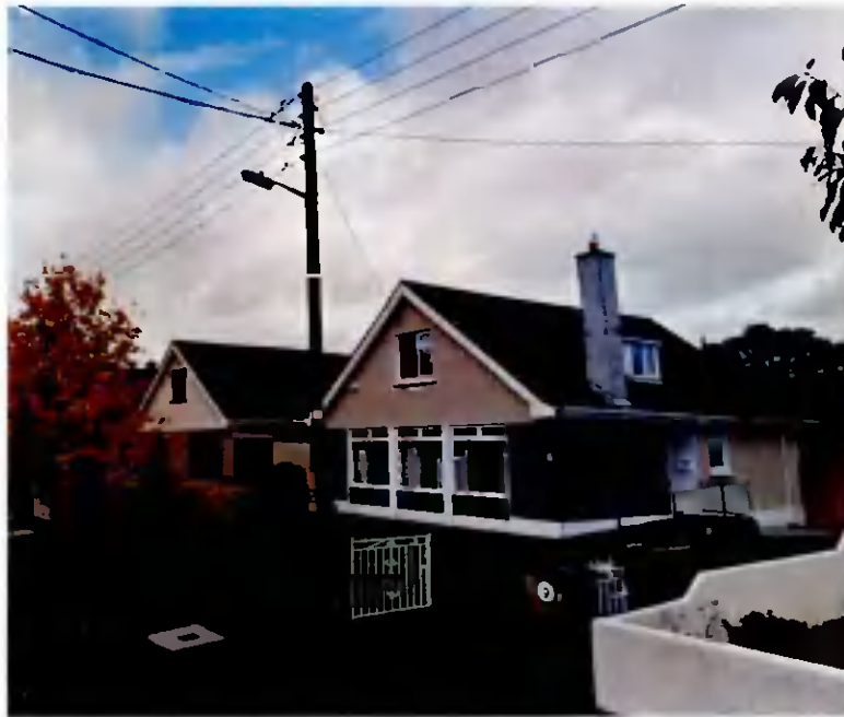
Figure 1.2 – Presence of Overheads lines at entrance
