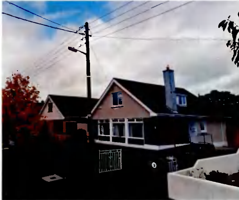
Figure 1.2 – Presence of Overheads lines at entrance
