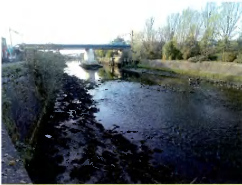
Plate 3.7 The River Tolka in the lower tidal reaches showing modification and retaining quay walls
