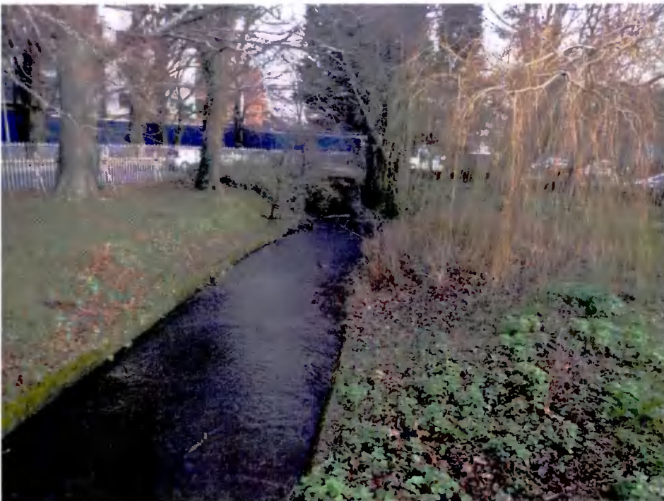
Plate 3.13 The River Poddle at Poddle Park showing heavy modification prior to underground culverting at Mount Argus Park
