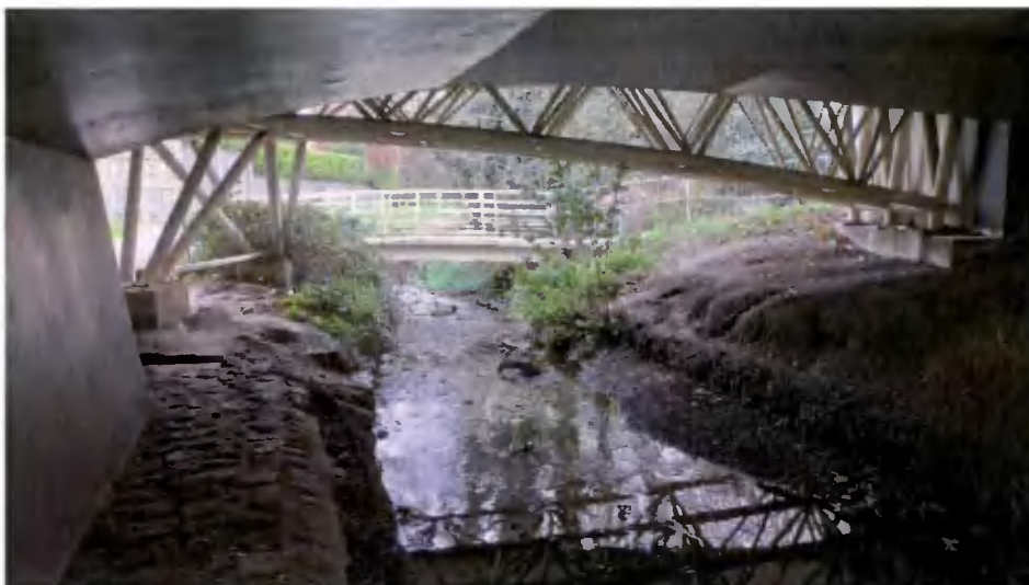
Plate 3.20 The Wyckham Stream upstream of the River Slang confluence along the Wyckham Way walkway
