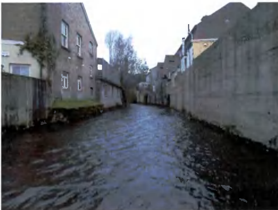
Plate 3.11 The lower River Camac at Kilmainham, heavily modified and bound by retaining walls
