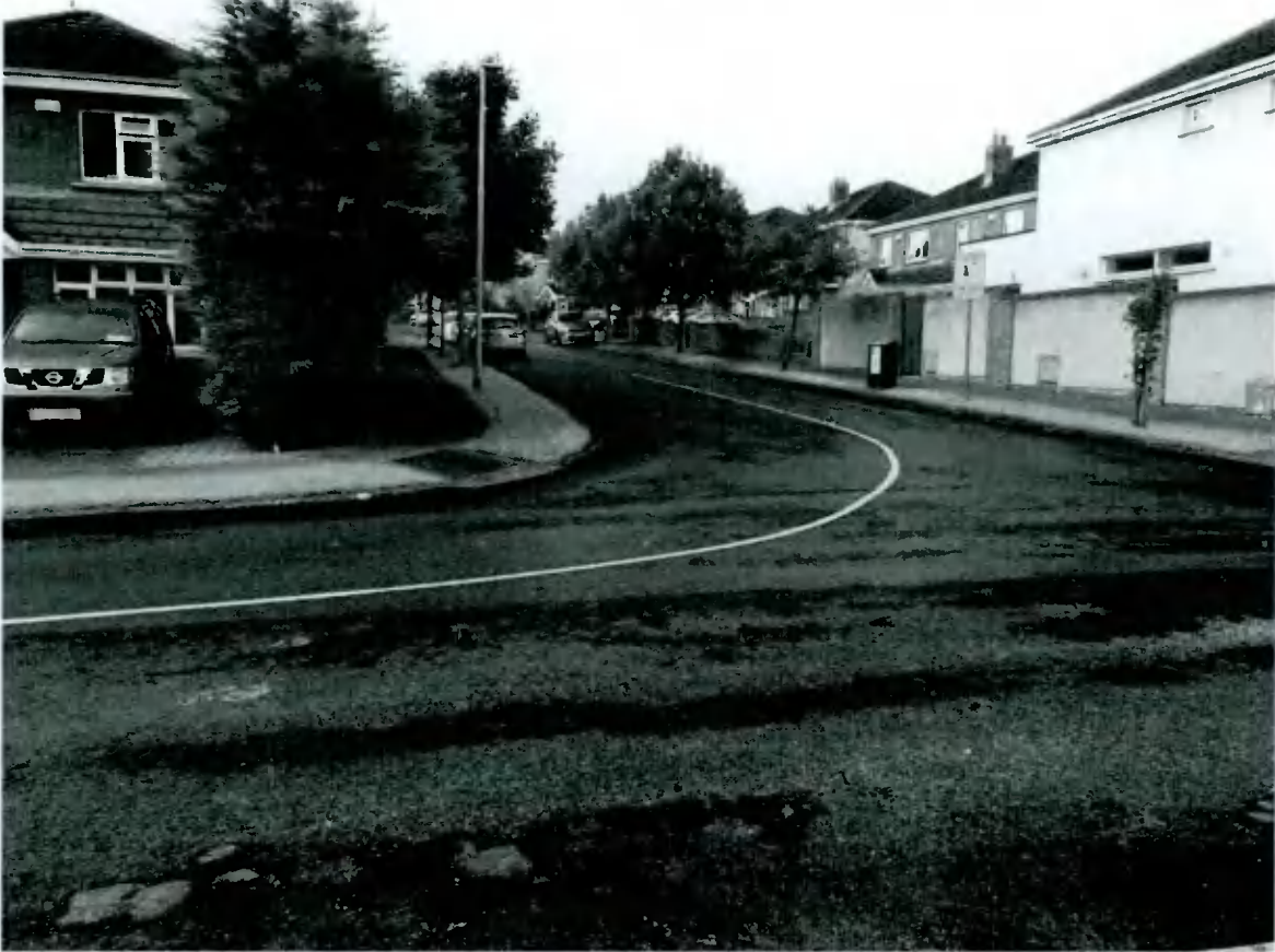
Appendix 6 - 90 degree corner at bottom of Grangebrook Avenue - blind corner
