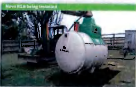
Novo RL6+ Wastewater treatment plant installed
