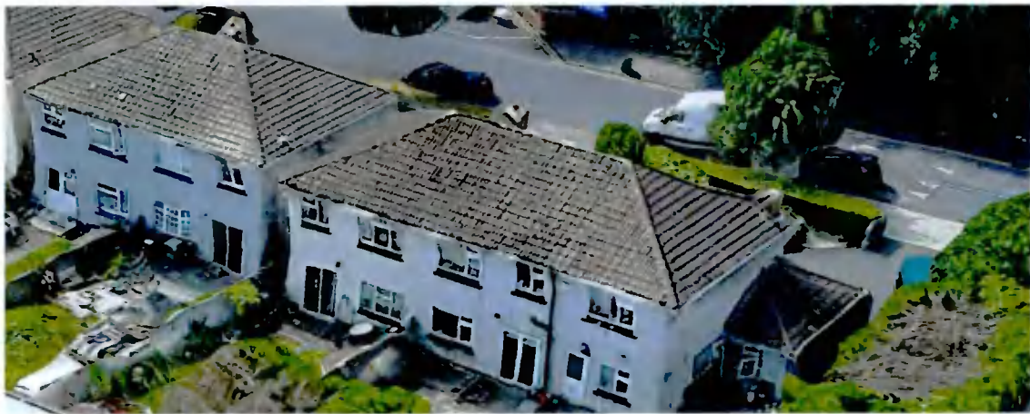
Figure 10: View of No.s 1 & 2 Oakcourt Ave.
