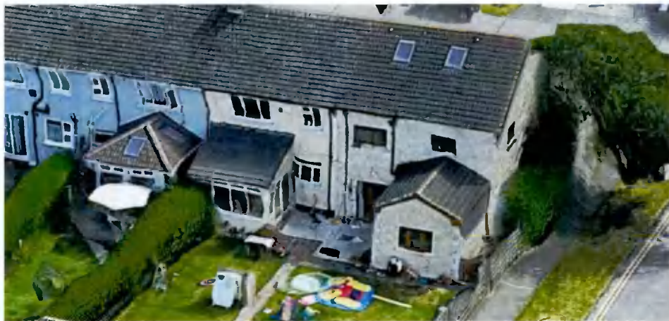
Figure 14: View of No.s 215 & 215A Palmerstown Ave
