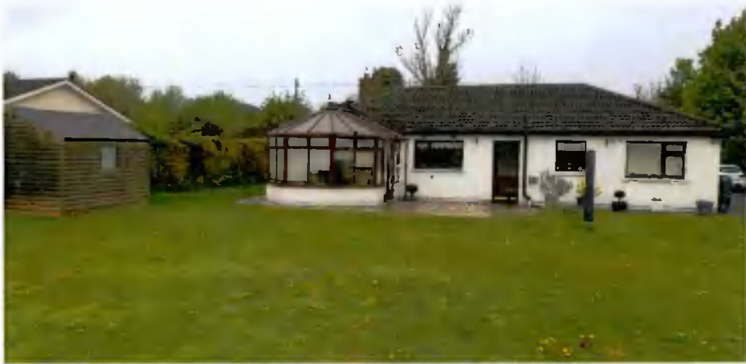
Fig. 1 Rear of existing Hawthorns Dwelling
