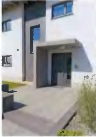
Fig.1 Example of the entrance canopy
