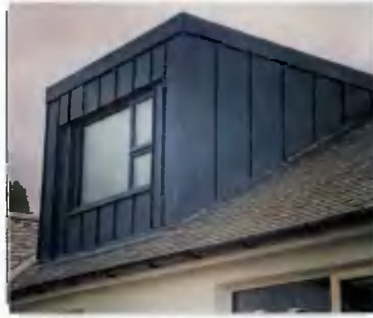
Fig. 2 Example of metal standing seam dormer roof
