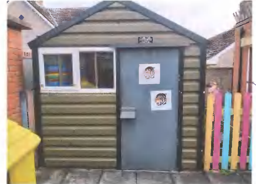
PICTURE OF EXISTING STEEL SHED FOR STORAGE
